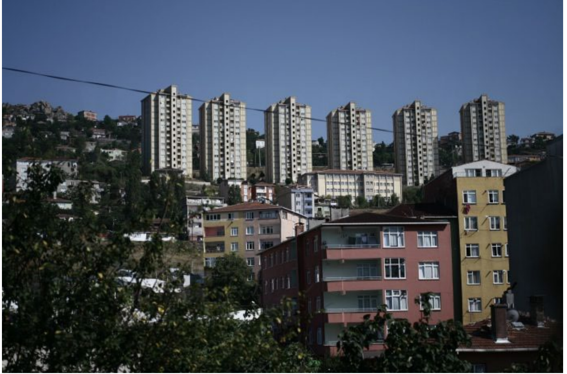
Figure 14, The Başibüyük construction site 28
