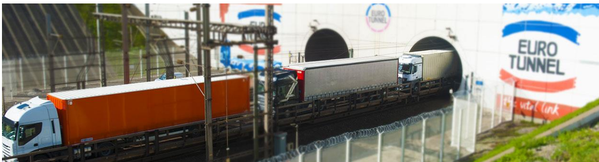
Figure 5.2 – Roll on - Roll off transportation in the Eurotunnel [45]
