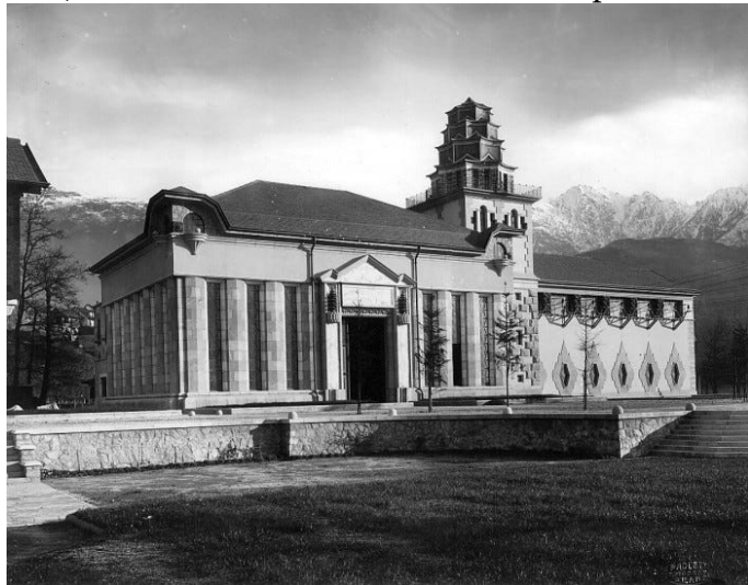
Image VIII.9: Power Plant of Creva d'Ossola, 1925
