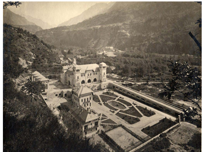
Image VIII.7: Power Plant of Verampio, 1910
