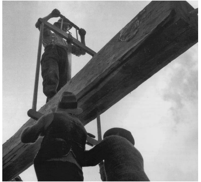
Image VI.5: Men constructing the Block Bau house
