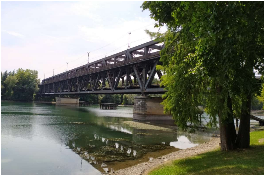
Figure 1: “Punt da Fèr”, Sesto Calende (Italy). Truss bridge on Ticino for trains and cars.
