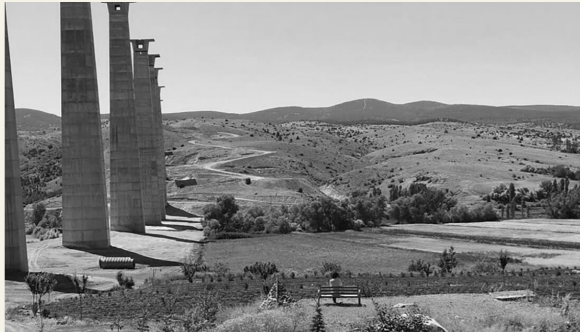
Images 77: View of the eco village Source: https://www.guneskoy.org.tr/Guneskoy
