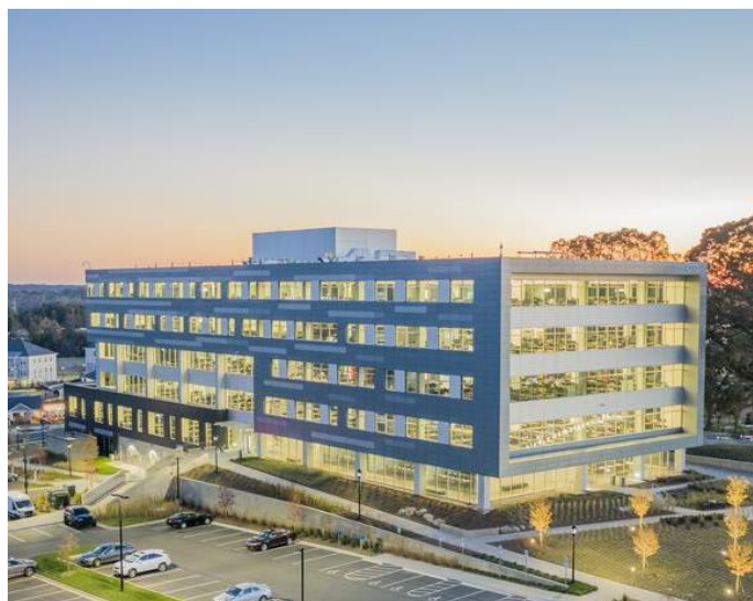
Figure 4.5: Corning Optical Communications HQ
