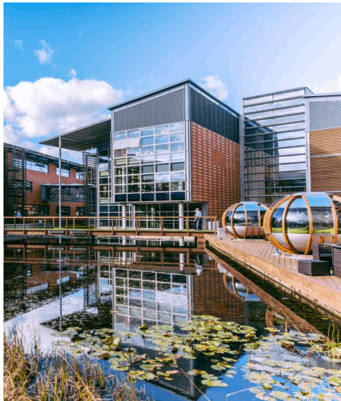
Figure 4.4: Vodafone Group Global Headquarters
