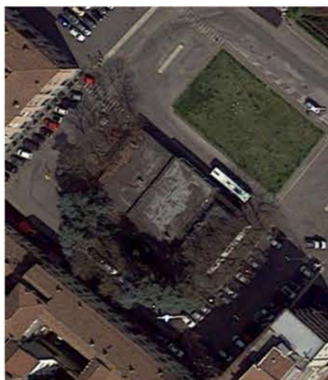
Existing satellite imagery of the abandoned bus station built in 1955.
