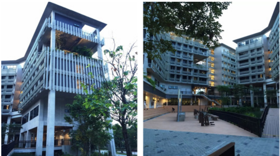
Figure 51: The green space in the building Source: Archigardener, 2015
