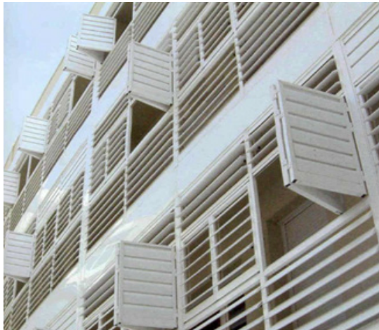
Figure 26: West elevation (courtyard): facade with shading by means of folding shutters and adjustable louvers
