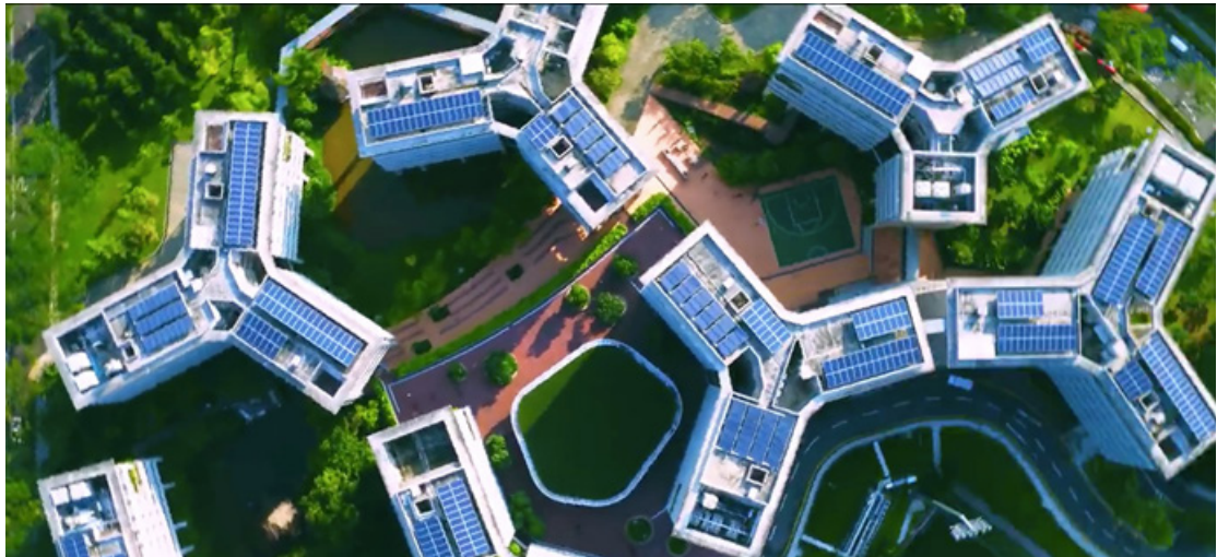
Figure 50: Solar panels on the roof Source: Archigardener, 2015
