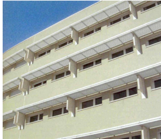
Figure 26: West elevation (courtyard): facade with shading by means of folding shutters and adjustable louvers
