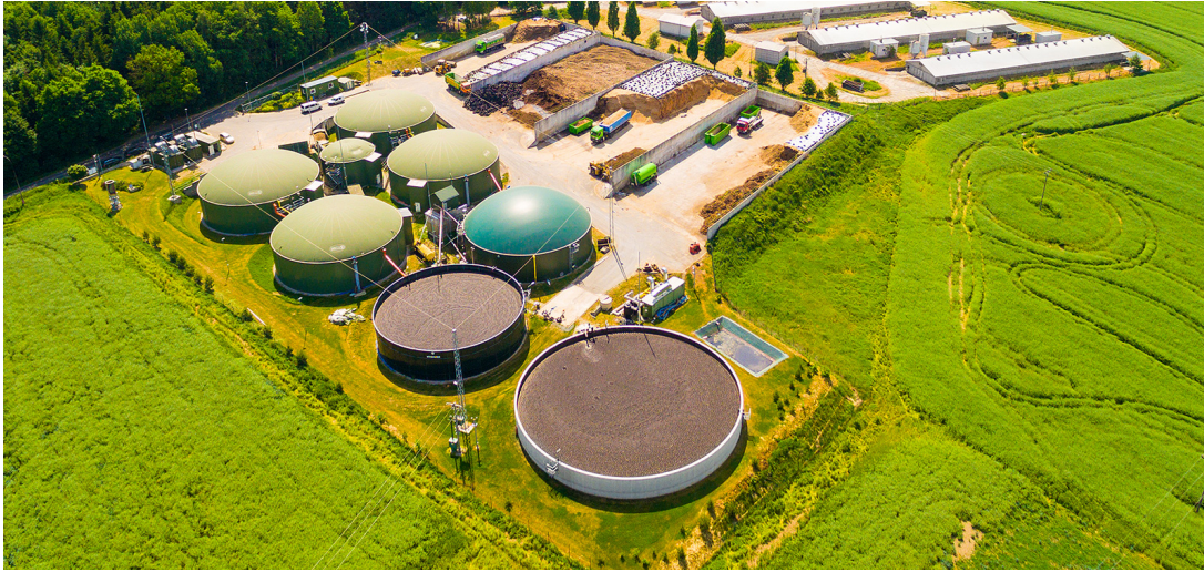
Figure 2.1: Aerial view of a biogas production facility, including basins for post-digestion and feedstock storage basins, [38].
