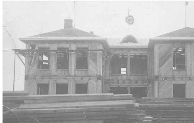
Primary school in the past
