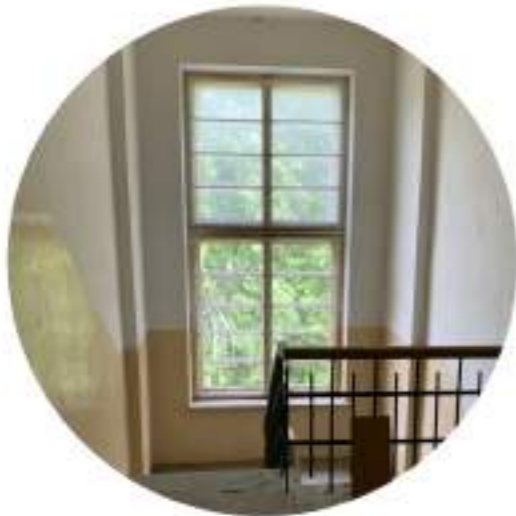
Bearing Exterior wall
