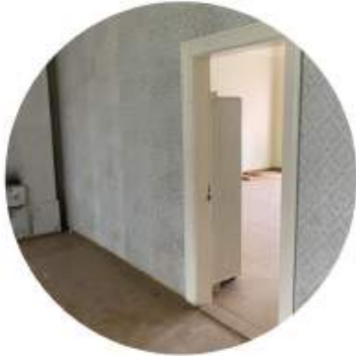
Partition Interior wall
