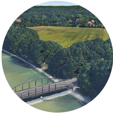
Fig.25. Site view from the south-west;
