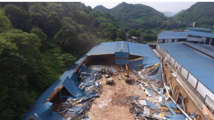
8. Demolish illegal factories
