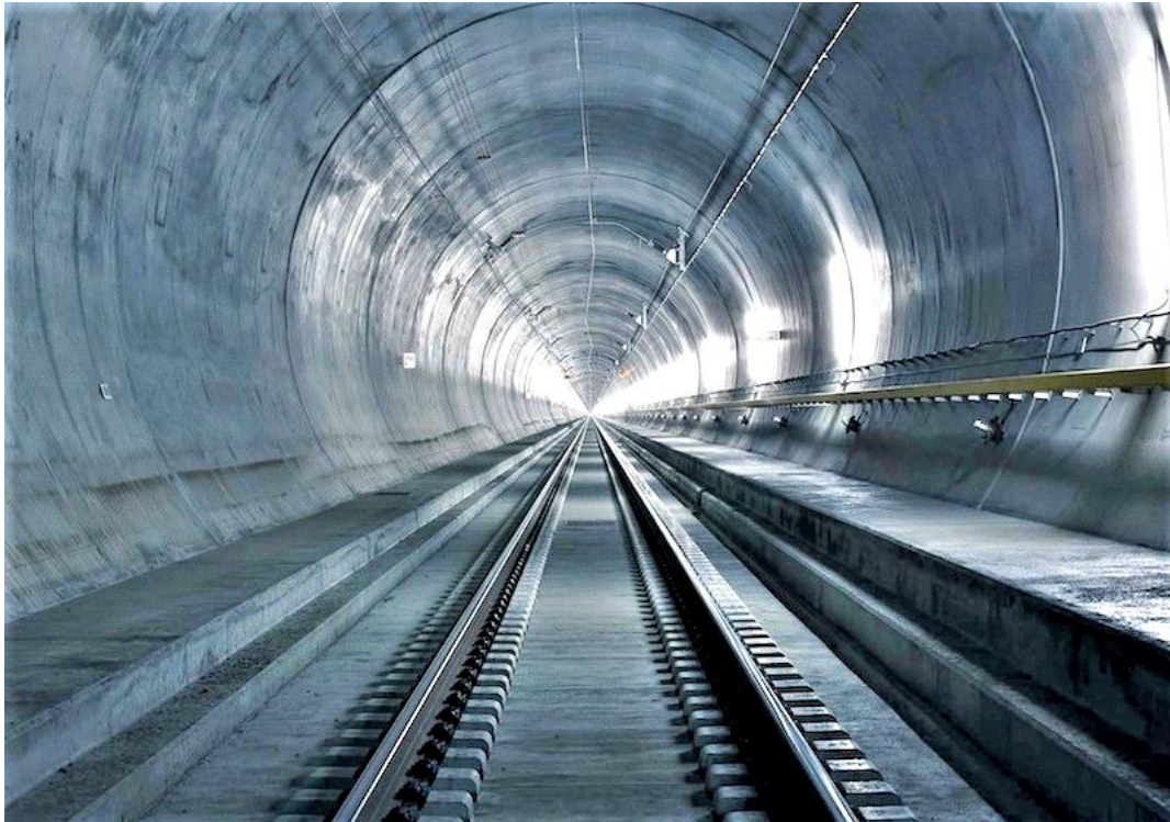
Figure 4-1: Rails anchored to a concrete slab. San Gottardo's tunnel - Switzerland
