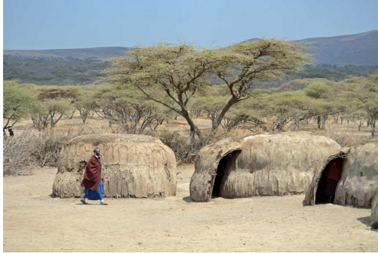
Figure 1.4: Traditional Maasai house (Enkang) made with dung mixed with mud and placed on a structure of flexible branches. The maximum height of the house is about 1,5 m. [6]
