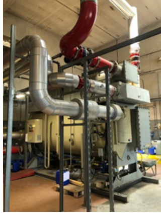
Figures 5-6: Primary system Absorption chiller
