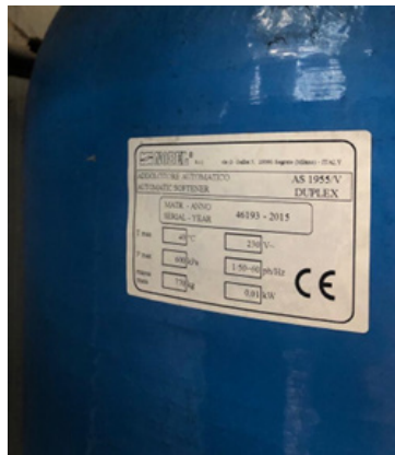
Figure 7-9 Primary system Softening system
