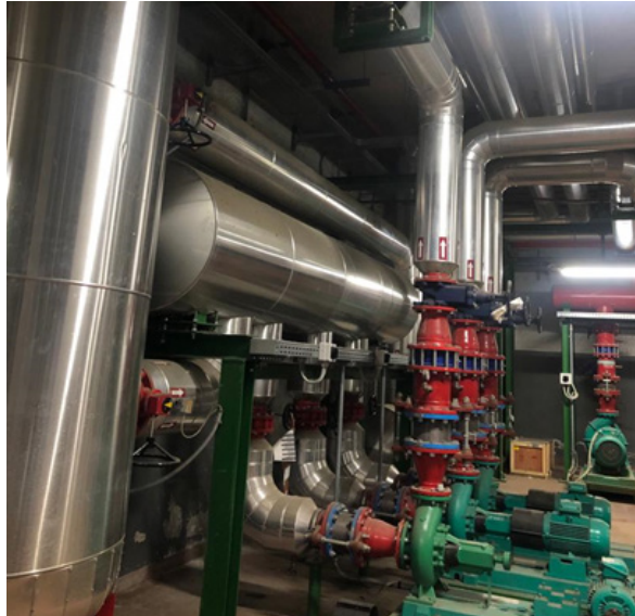
Figures 10-11: Primary system pumping station and heating exchangers
