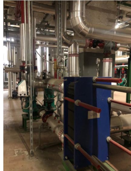
Figures 10-11: Primary system pumping station and heating exchangers
