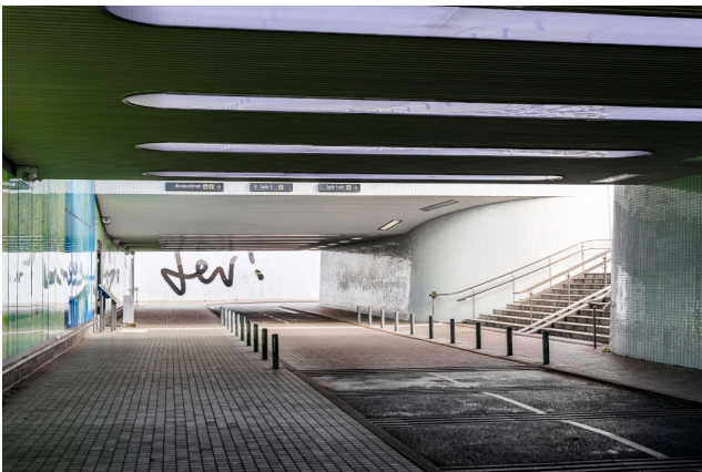
Fig. 5 Tunnel with open spaces, wide bike and walk lanes, an intermediate alternative exit, round corners and optimal light flow
