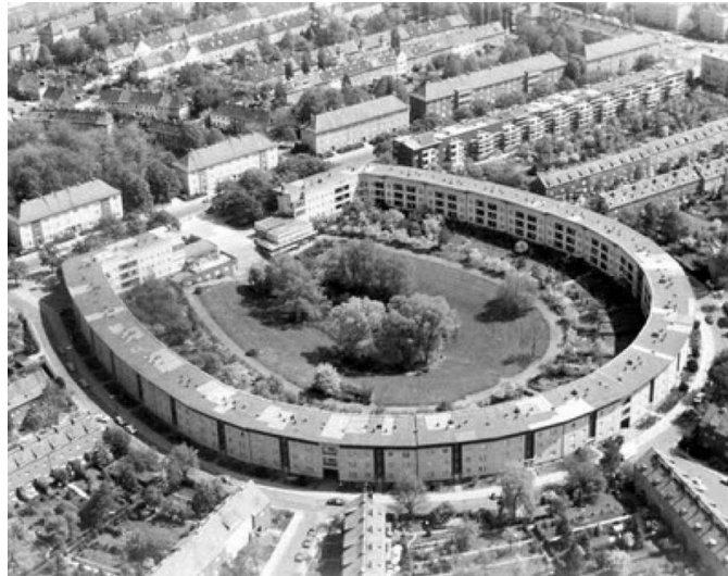
Figure 3. Bruno Taut, Britz Horseshoe Estate, 1922 http://architectuul.com/architecture/view_image/britz-horseshoe-estate/488
