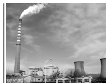
Wuhai Thermal Power Plant
