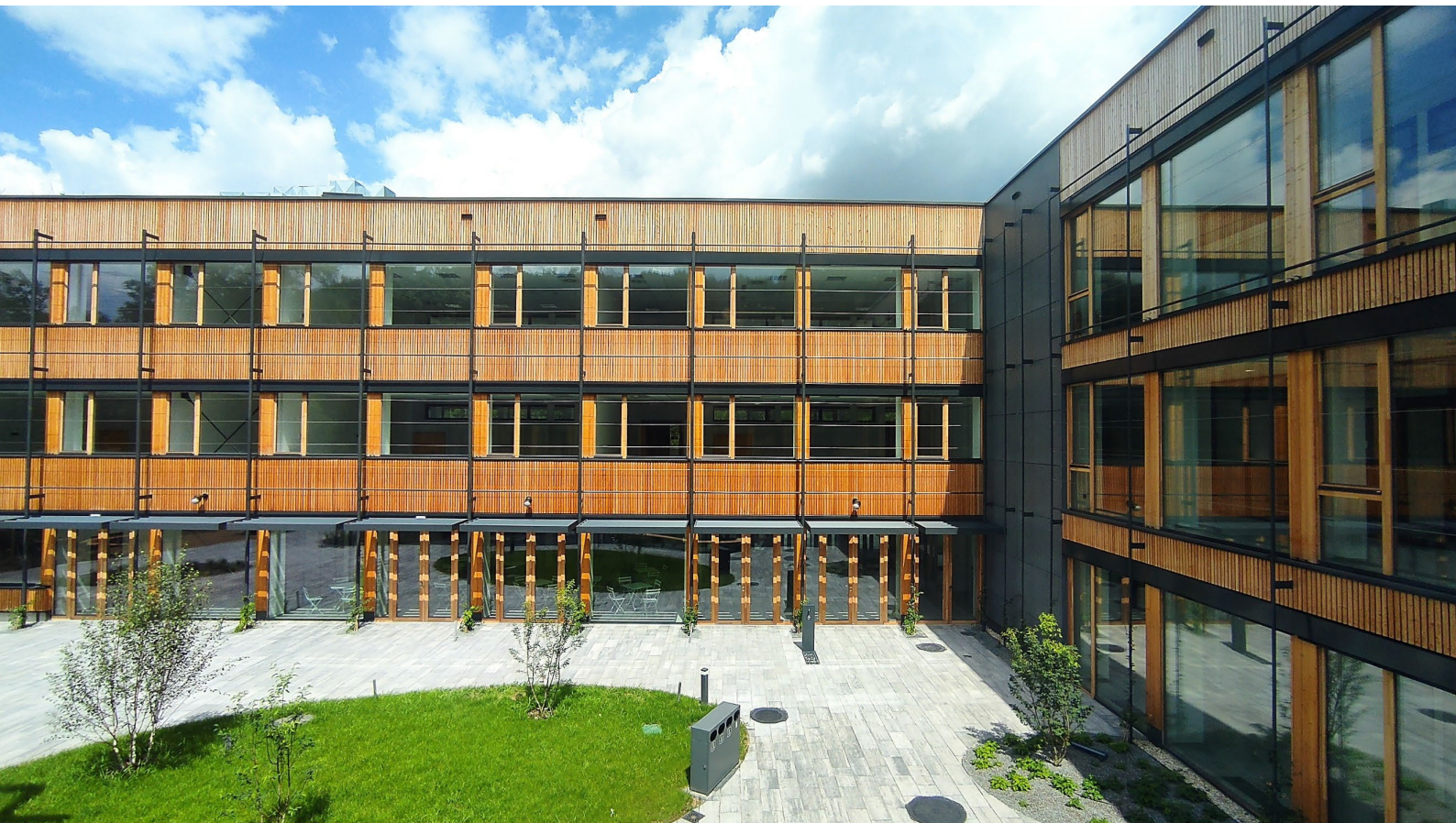
Figure 75: Revitalization into a smart, safe, sustainable, energy and carbon positive high school building. ENVILOP, wooden facade developed at CTU, 2022, Prague
