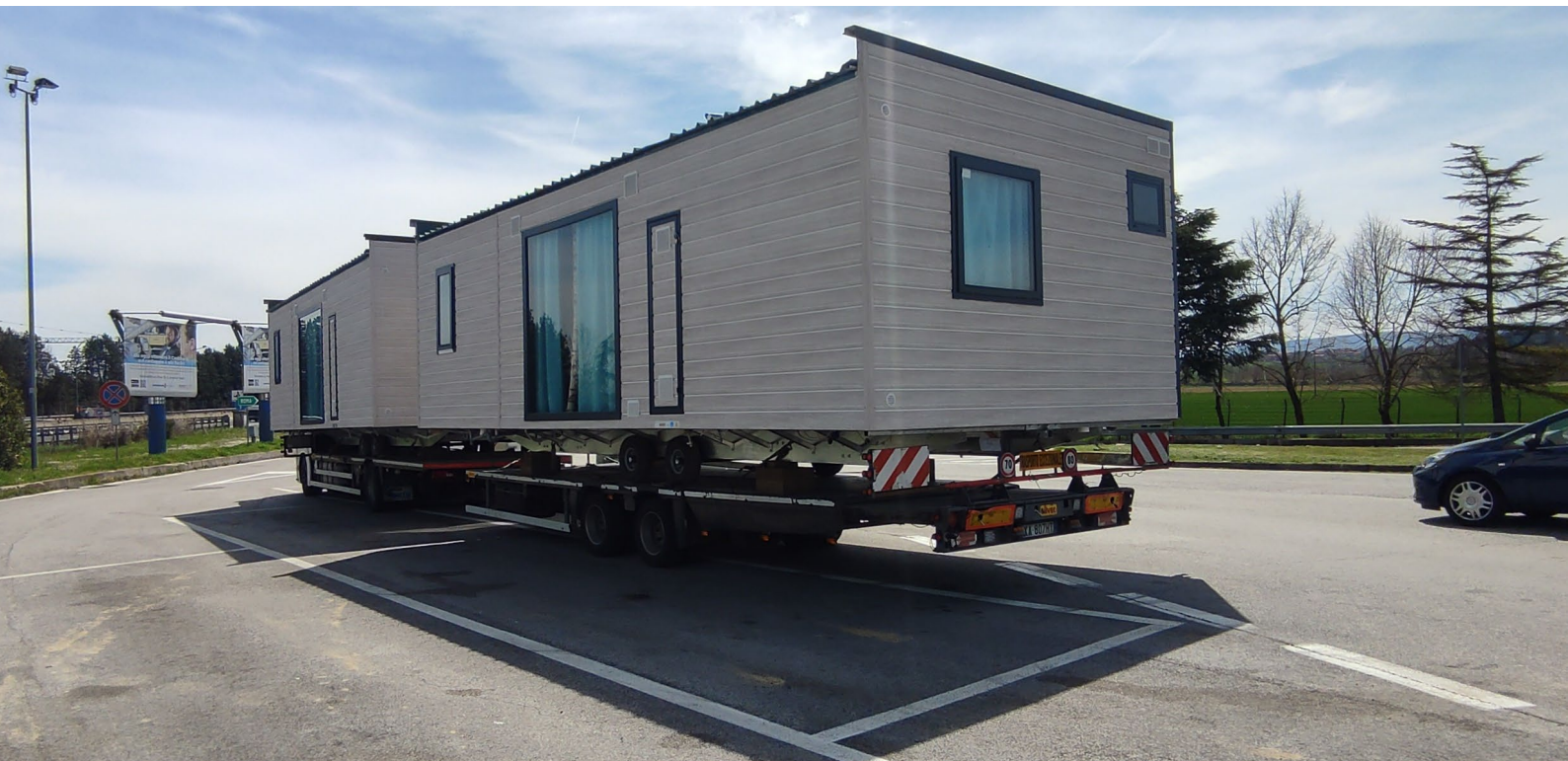
Figure 80: 3D Housing Module truck carrying
