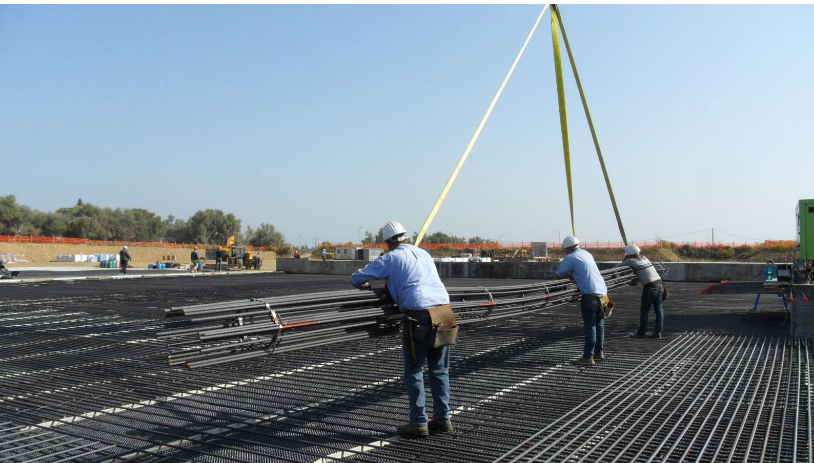
Figure 45: Reinforcement Steel Mesh Carpets
