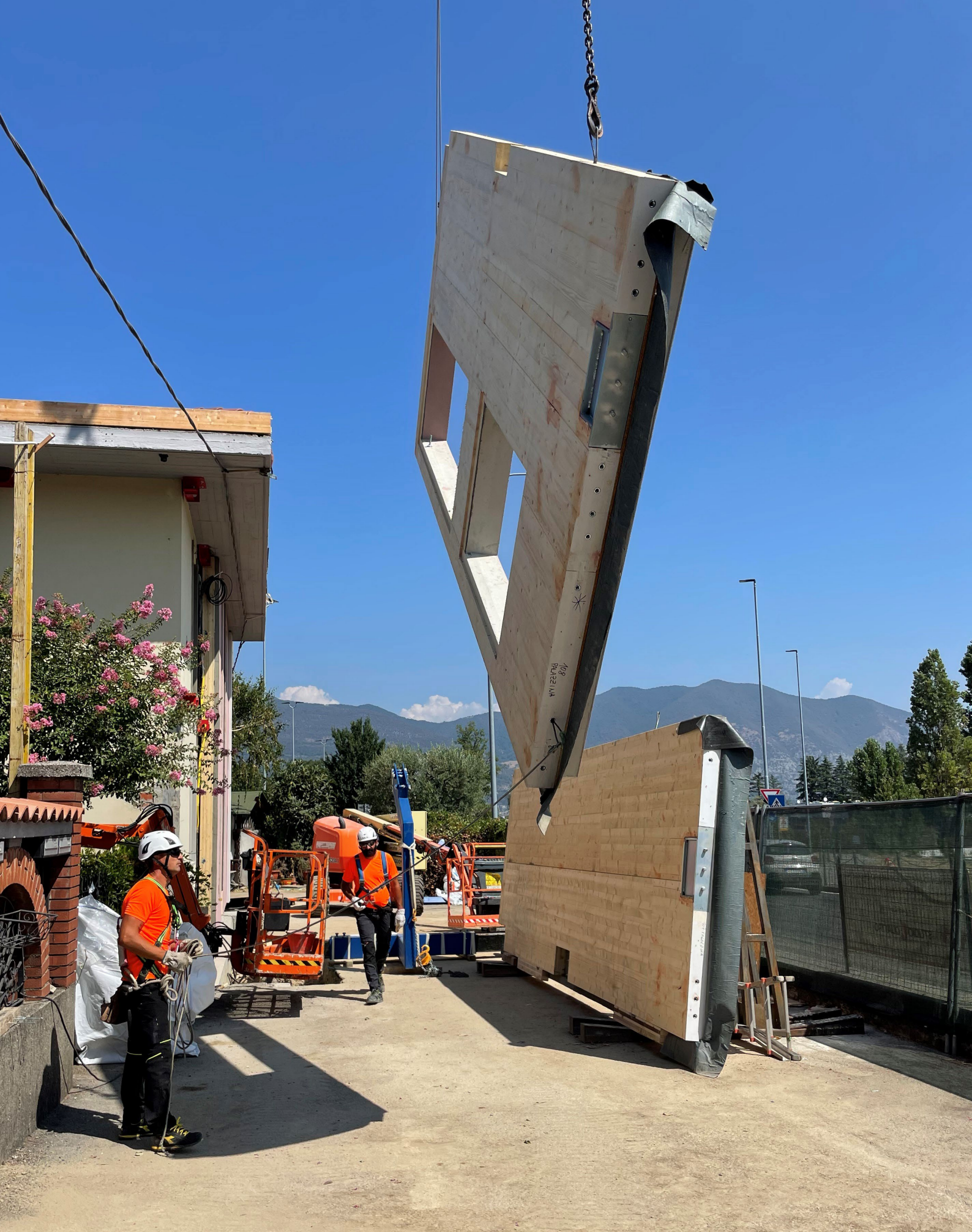
Figure 125: Existing Building Refurbishment by Panelization, Corte Franca (BS), Italy [Edera]
