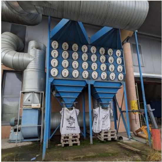
Figure 83-3.2 Dust Filters (Liudmila Sidorova, 2023)
