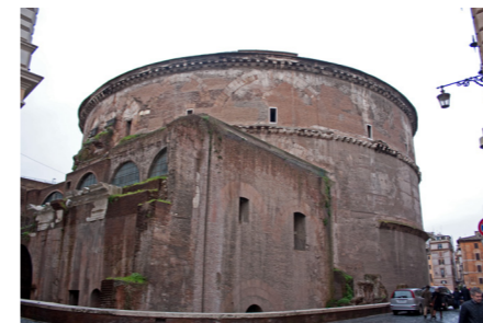
Figure 17: exterior of the rotunda.
