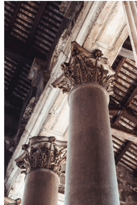
Figure 15: detail of the column. Moritz Kindler, Rome, 2020.
