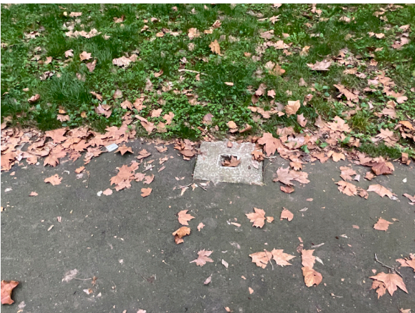
Figure 11. There are also concrete blocks embedded in the ground at the edge of the rubber paving. Source: Taken by the authors
