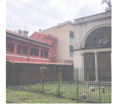
Buildings affecting the visual experience
