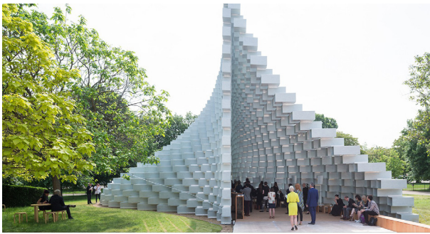
Figure 5. The Serpentine Gallery 2016 was designed by BIG, using wood and fiber glass. Eco-friendly, lightweight materials and unique design are the prerequisites for this structure to be presented in the historic garden. Source: https://diariodesign.com/2016/06/serpentine-gallery-2016-por-big
