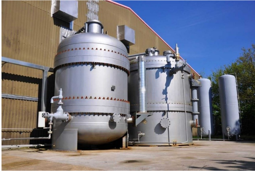
Fig. 2.11: Small scale pilot plant made by the new National Facility for Pumped Heat Energy Storage
