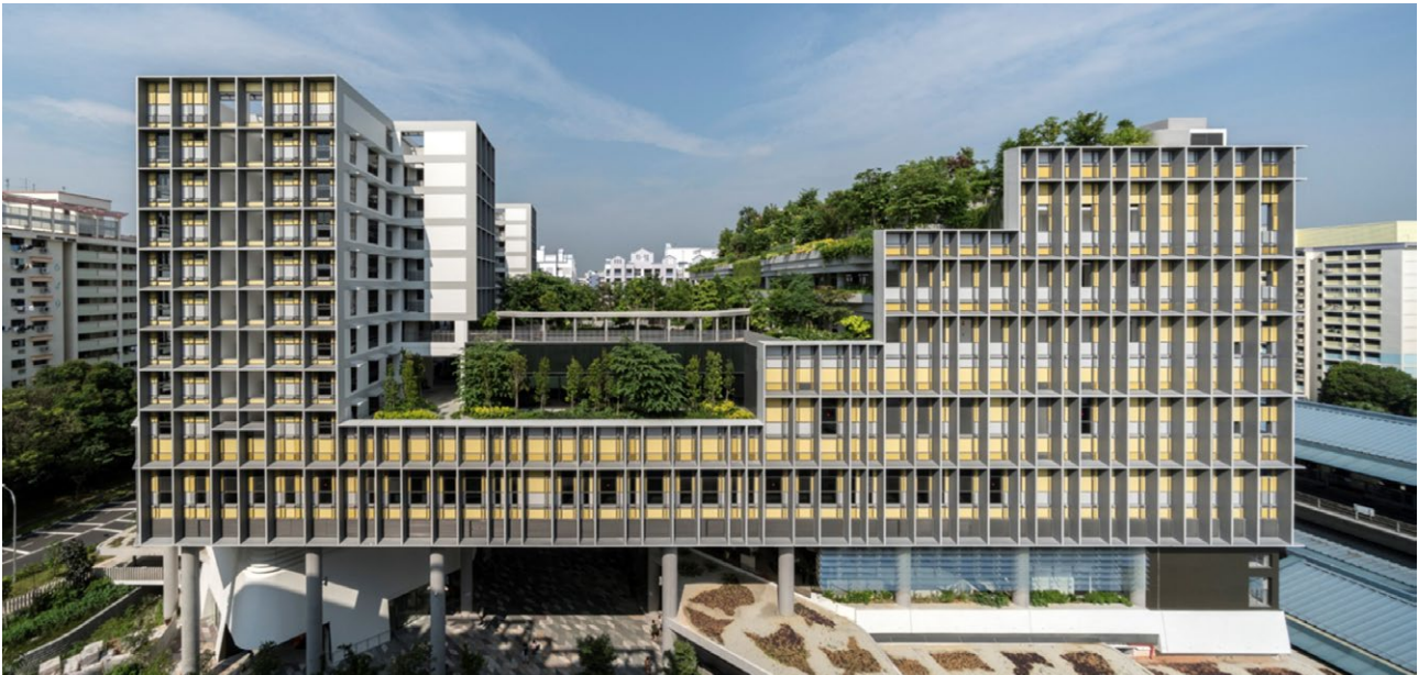
Figure 69. Exterior view of Kampung Admiralty, highlighting its mixed-use vertical organization and integrated greenery. (WOHA Architects, 2018.)
