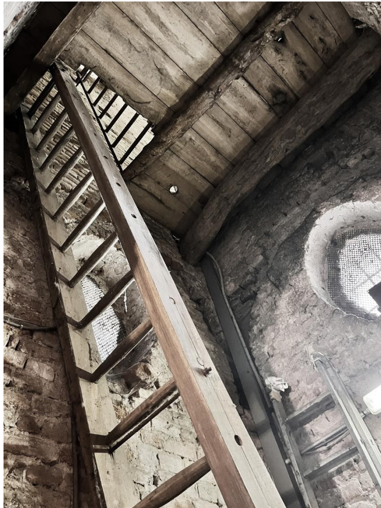
Figure 8 - Interior of the bell tower
