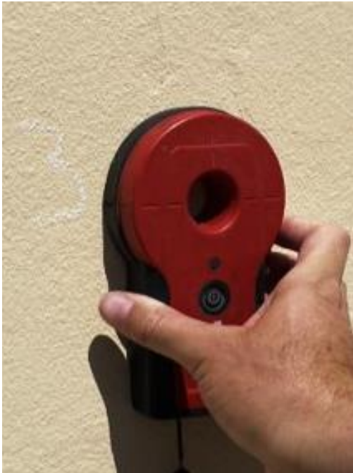
Figure 32 – Photographic representation during in situ testing
