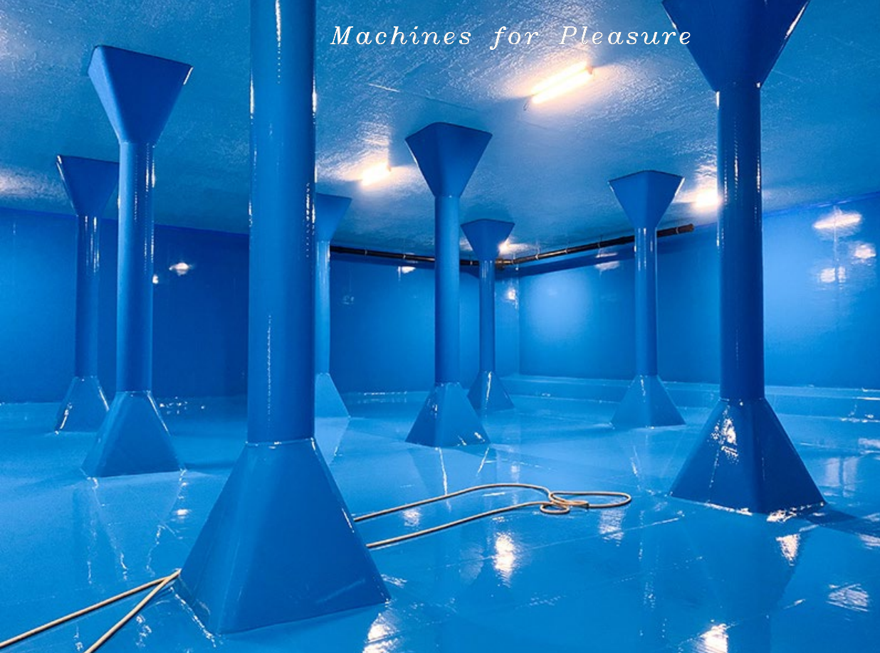
Image credit: ZurichStadtWasser, archive, 2018.
