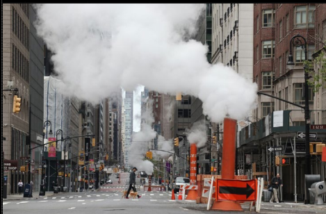
The clouds of steam rising from New York City's street grates , in this picture by Jan Hosling of 2022, powerfully reveal what normally remains invisible. Beneath the asphalt lies a dense network of pipes, ducts, and infrastructure that transport energy, heat, and materials: an underground world brimming with potential.
