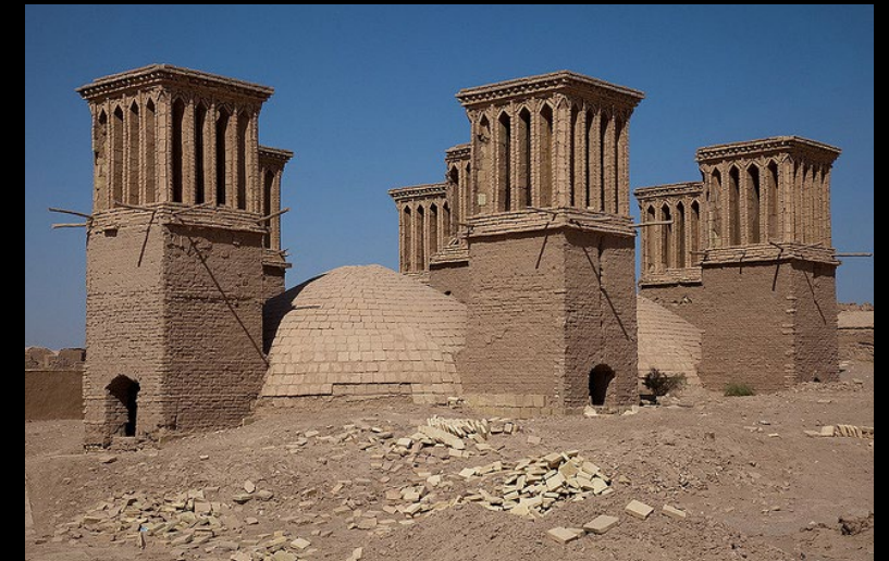
Badgir (wind towers) in Yazd, Iran, a historical example of passive engineering. These structures, dating back centuries, were used to ventilate and cool buildings in hot, arid climates.
