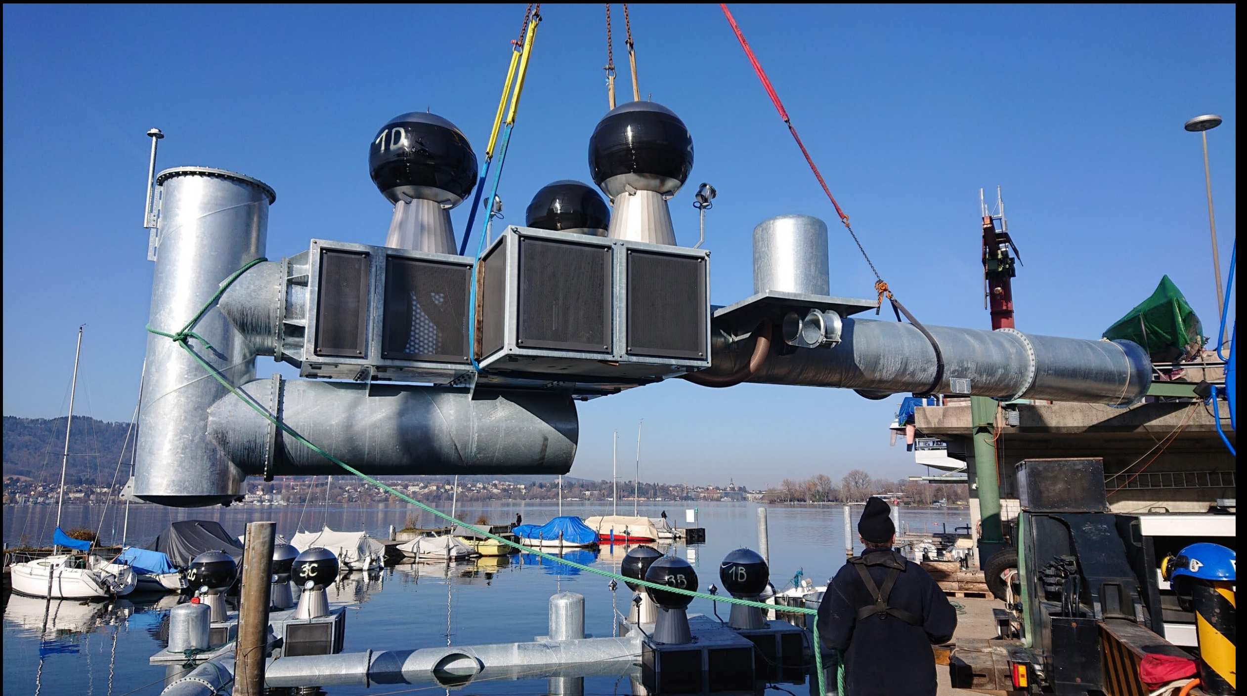
Aquoretum, installation in progress, ETH Zurich, c. 2020. Credit: Aquoretum, ETH Zurich.
