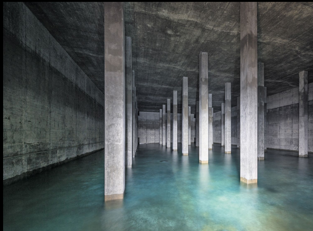
Archival images of Zurich underground water reservoirs, copyright Stadt Zürich Wasserversorgung, 2015
