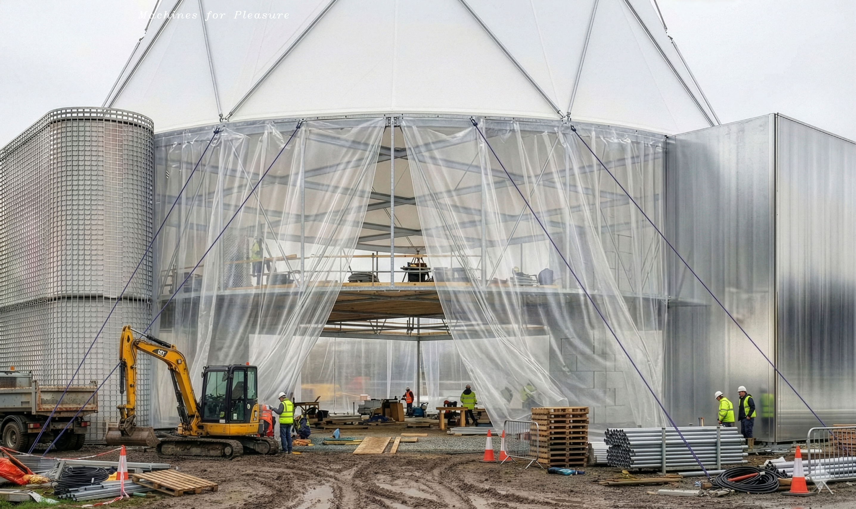
Constructive process - a series M/ Josefstrasse Zentrale
