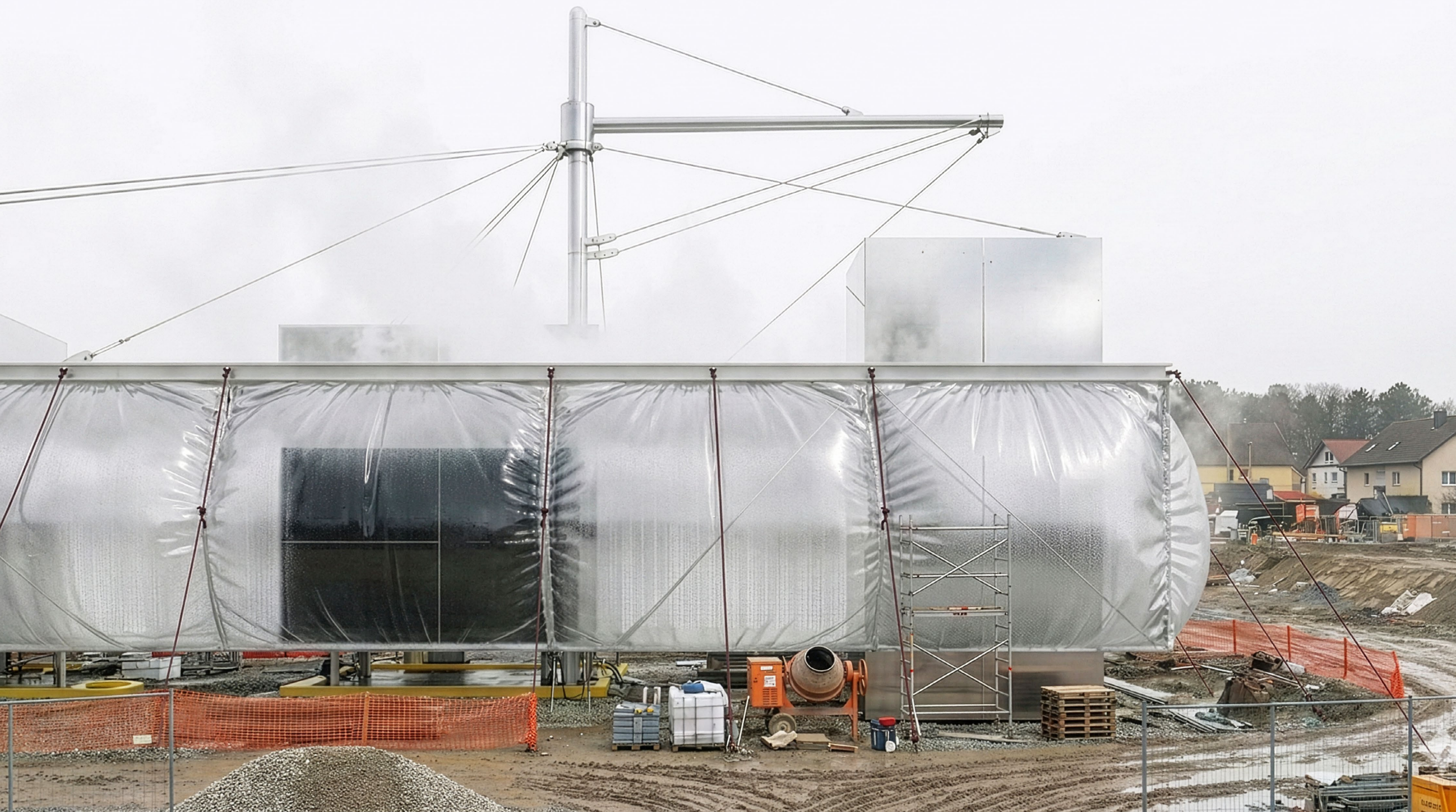
Constructive process - a series L / UntererLetten
