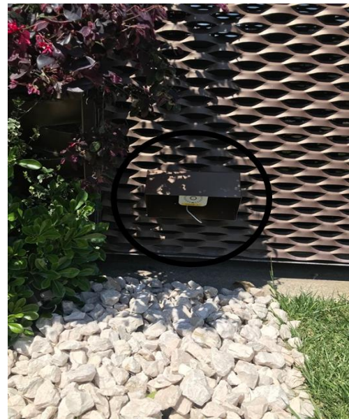
Figure 167: Sensors installed on the Green Panels in Brescia, ItalMesh Headquarter
