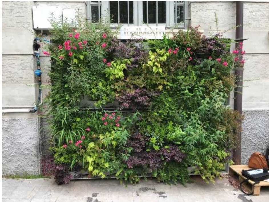
Figure 30: Case study 1 Building 9- Green panel
