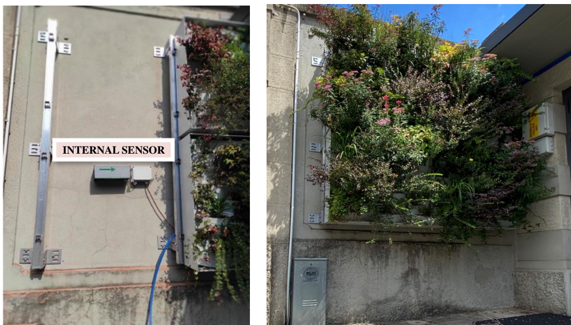
Figure 68: Case study 2 building 10- Green panel mounted on the wall
