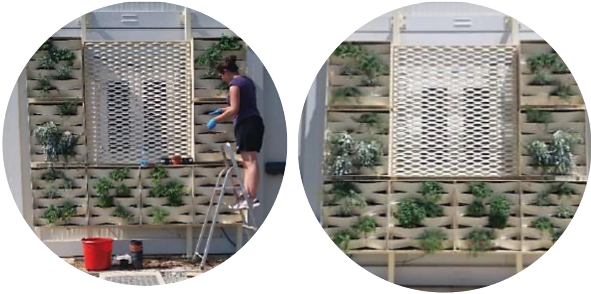
Figure 117: Installation of Green panels in Cyprus Institute
