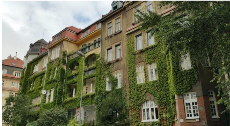
Figure 6 :Applying of Direct Green Facade on Bratislava Slovakia building (Pixabay, 2016)
