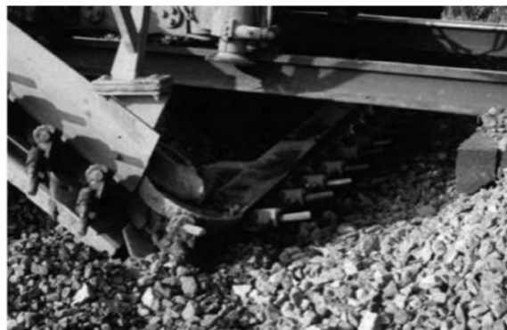
Figure 18. The undercutting operation (Li, Hyslip, Sussmann, & Chrismer, 2015).
