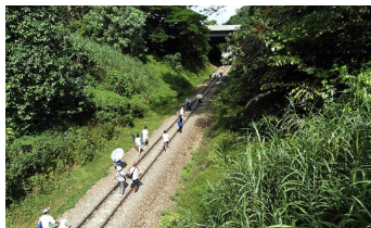
On ground railway voids
