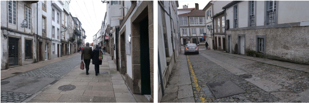
Figure 3.7: Picture of the paving of a road in the historical centre of Santiago de Compostela, Spain. It is interesting to note that also in this case different pavings are used for different urban elements: sidewalks and roads, that are on the same elevation.
