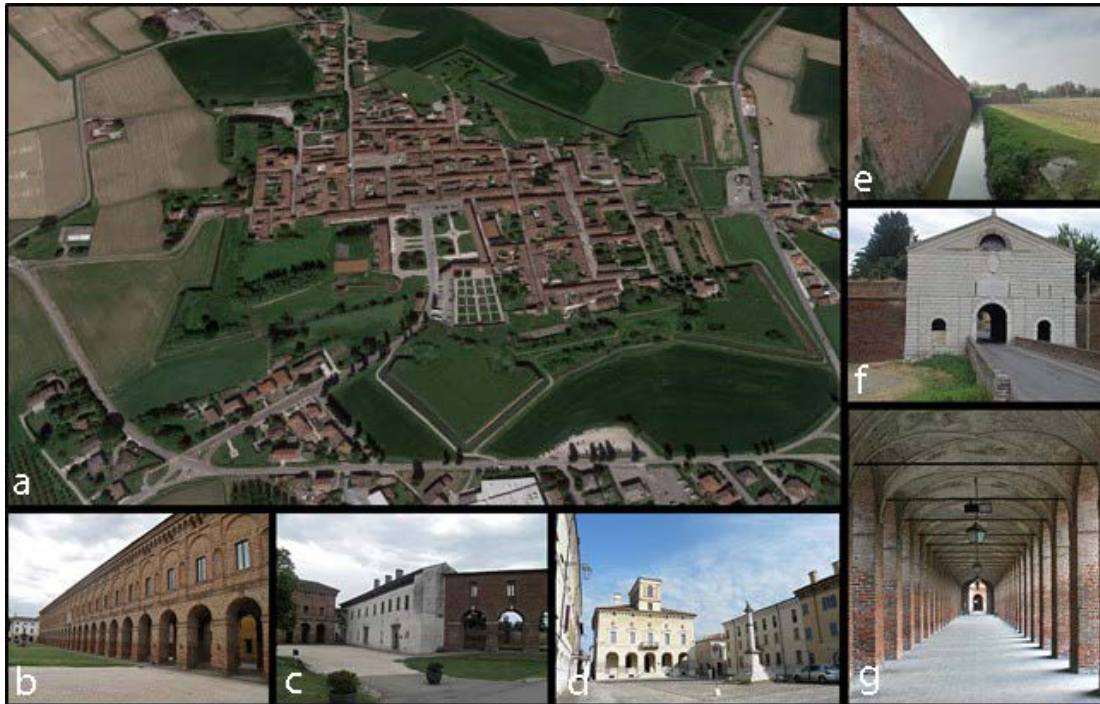
Figure 3.1: Some photos of the case study: the historical city of Sabbioneta, which is a Unesco site together with Mantova. a: a bird's eye view of the city, the city centre and the fortified walls with the peculiar shape. b: the Galleria degli Antichi facade on Piazza d'Armi. c: the main facade of Palazzo del Giardino. d: Piazza Ducale, with on the background Palazzo Ducale. e: one of the fortified walls, seen from outside the city. f: Porta Imperiale, one of the entrances of the city. g: the ground floor of the Galleria degli Antichi, which is a porch with cross-vaults and pillars.
