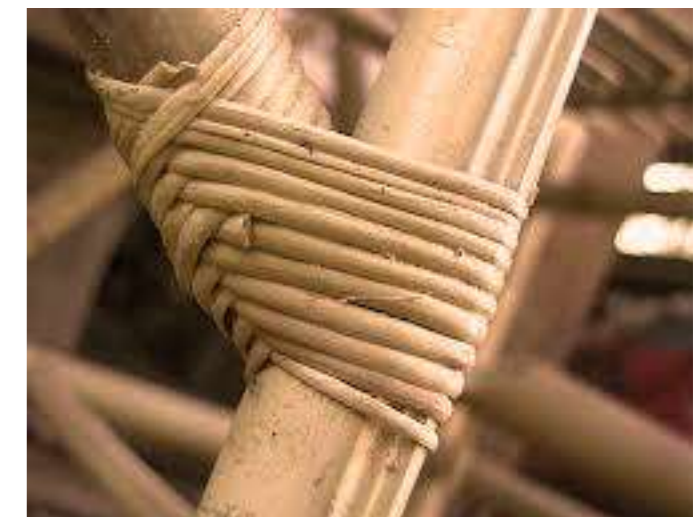
Figure 4-1 bamboo connection
