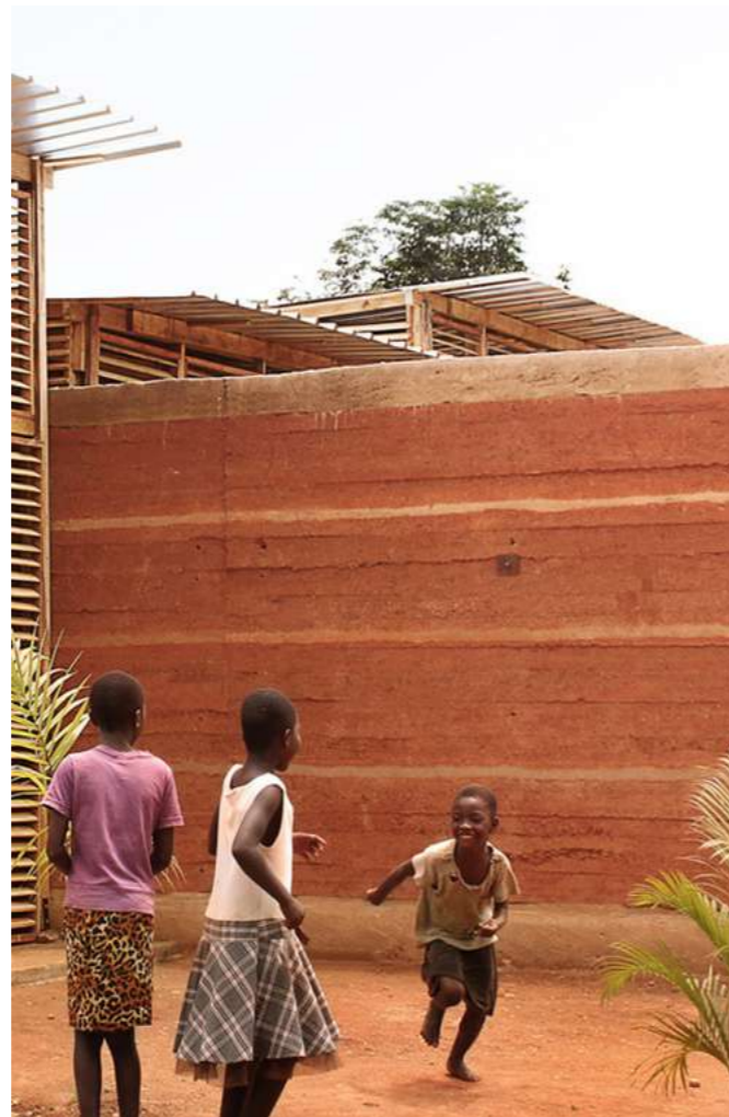
Figure 1.17 Rammed earth material in african house
