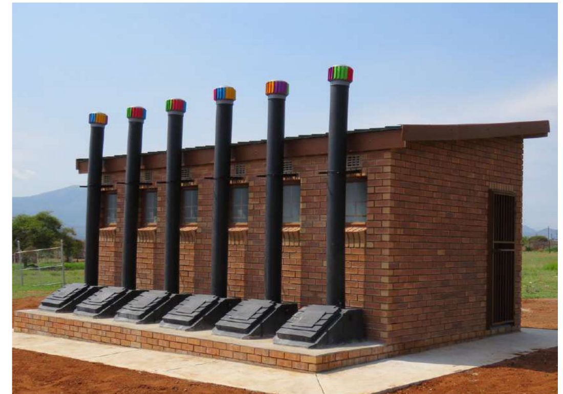
Figure 5.10 waterless toilets construction
