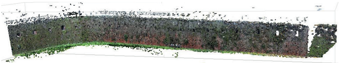
Figure 5.2.3.i Dense cloud obtained by photogrammetry of a portion of the moat.
