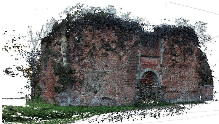
Figure 5.2.3.l Dense cloud obtained by photogrammetry of the exterior of Porta del Soccorso.
