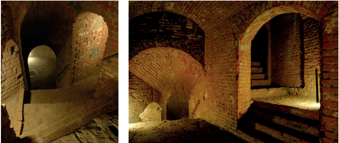
Figure 4.3.i-l The entrances to the three casemates inside Torre della Colubrina. Photo from the website http://www.milaneicantieridellarte.it .
