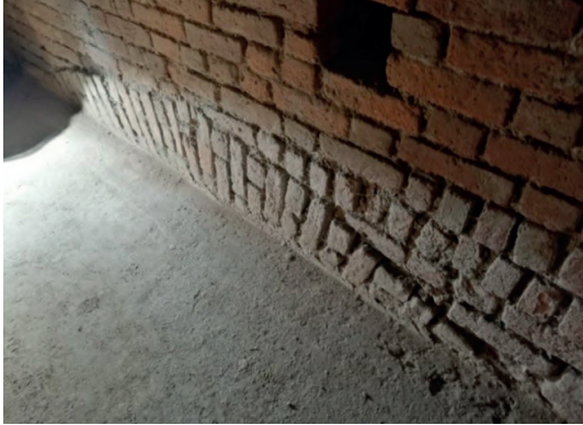
Figure 5.6.1.e One of the arches on the inner wall of the counterscarp passageway.
