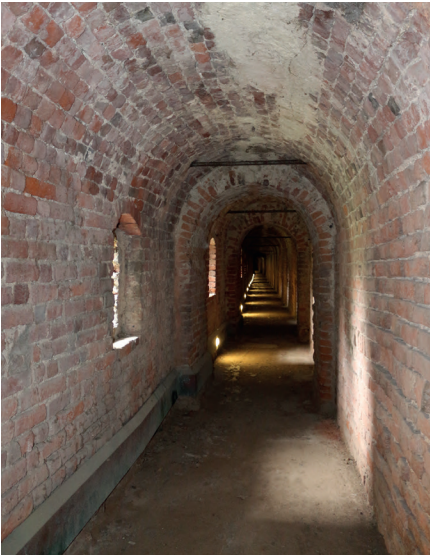
Figure 4.3.g A section of the counterscarp tunnel.
