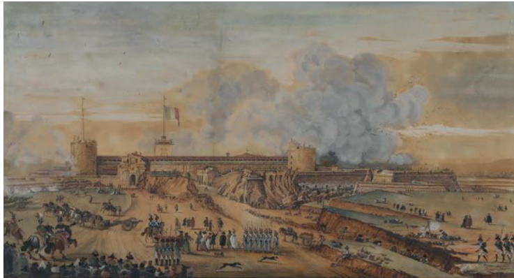
Figure 4.2.n Picture of the demolitions at the Castello Sforzesco ordered by Napoleon Bonaparte. C. first year of 1800. Document in the Civic Historical Collections (Milan).
