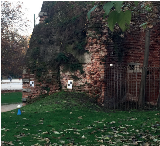
Figure 5.3.2.l-m Detail of the wrong surface processing, adjacent to Porta del Soccorso (I). Image of the real shape of the ground in this area (m).
