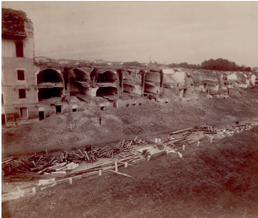
Figure 4.2.q Photo of the demolition phase of the Ghirlanda, during the restoration of the castle. 1893. Document in the Civic Photographic Archive (Milan).
