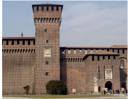
Figure 4.2.d Tower of Bona di Savoia today.
