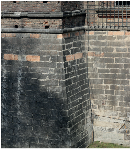
Figure 4.2.c Some areas where the castle shows signs of reconstruction, perhaps associated with the post-Republican period. The first one shows the transition from the use of stone to that of bricks, coinciding with the junction between the older and the later nucleus. In the second one there is an example of the reuse of stone blocks.
