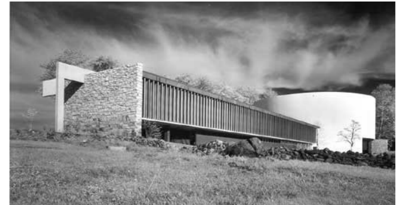
FIG. 38 - Cyclorama Building, Gettysburg National Military Park, by Richard Neutra, 1962
