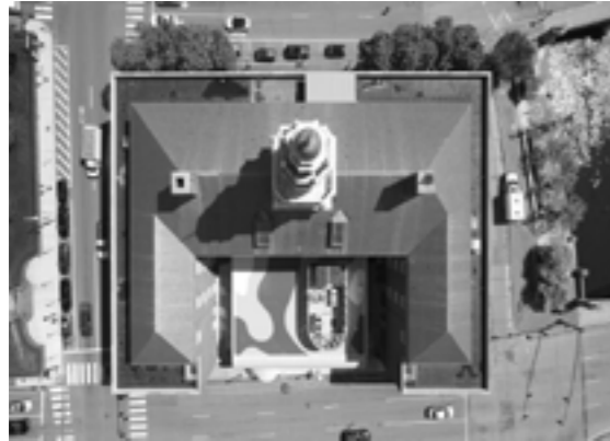
Figure 18: Building top view
