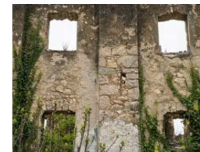
Figure 27. Limestone wall, exterior facade.
