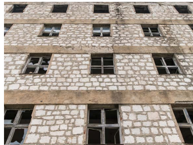
Figure 61. Magazine 7, southern facade detail. Note. Author's photograph.
