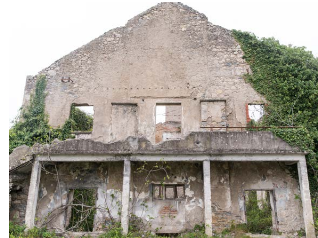
Figure 57. Magazine 5, east facade. Note. Author's photograph.
