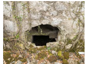
Figure 51. Basement level of Magazine 7, identified on site and added to the author's documentation, as it was not included in the original survey drawings.
