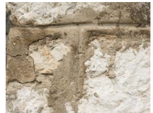
Figure 39. Cement mortar, Magazine 7
