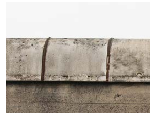
Figure 35. Steel bridge roof covering. Note. Preserved metal roof covering of the bridge between warehouses, consisting of galvanized steel sheet.
