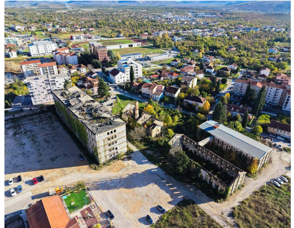
Figure 20. Aerial view of the Tobacco Station from the northwest. Photograph: Michel Beara, 2025. Source: private archive.
