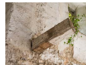
Figure 44. Timber beam imprint in masonry wall Note. Trace of the original timber floor beam embedded in the load-bearing wall.
