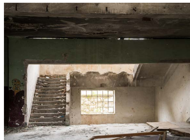
Figure 63. Magazine 7, interior staircase. Note. Author's photograph.
