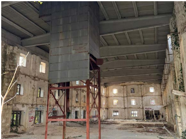
Figure 54. Magazine 2, interior view with original steel lift and later interventions. Note. Author's photograph.
