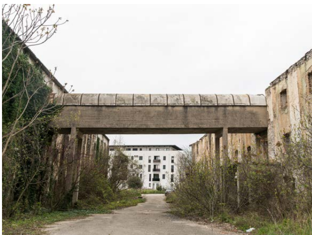
Figure 55. Bridge between Magazines, 1970s addition. Note. Author's photograph.
