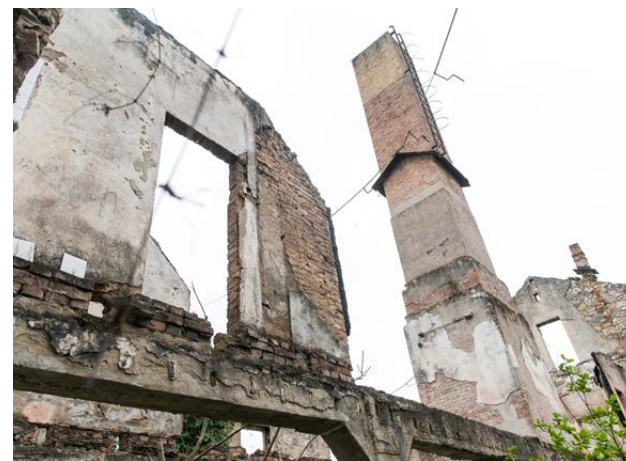
Figure 58. Magazine 5, interior view. Note. Author's photograph.
