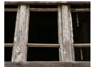
Figure 31. Timber window frame, Magazine 2
