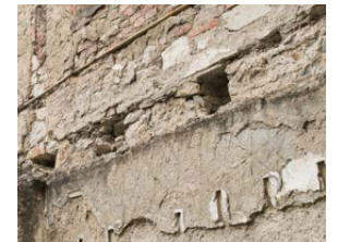
Figure 48. Beam pocket in masonry wall, Magazine 5. Note. Recess in the masonry wall used for embedding a timber floor beam, indicates the position of the original floor structure and represents a distinct feature of the masonry phase.
