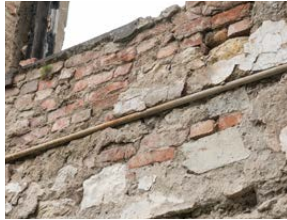
Figure 29. Clay brick composed wall, Magazine 5
