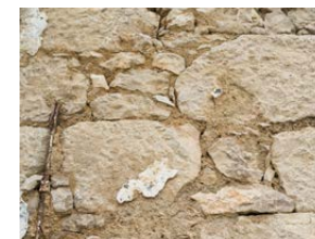
Figure 28. Limestone wall detail
