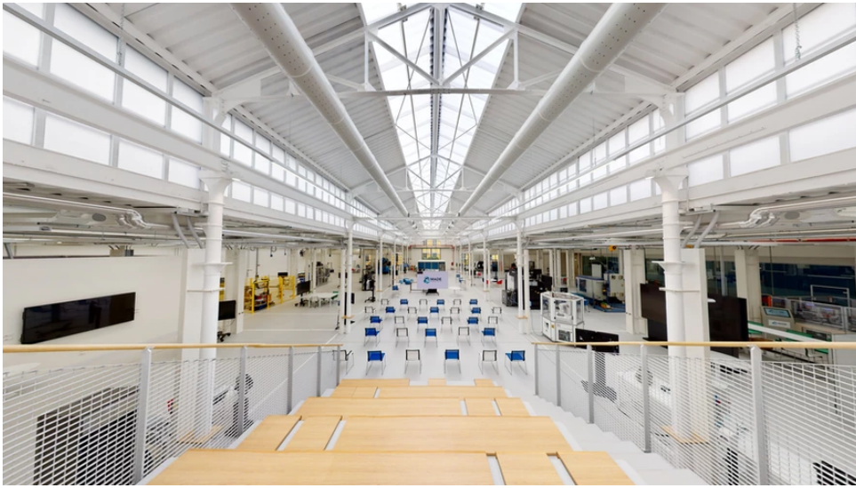
Figure 4.2: MADE building, Politecnico di Milano, campus Bovisa, inside.
