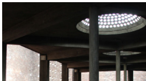
fig 4.98 Interior view seeing the cupola
