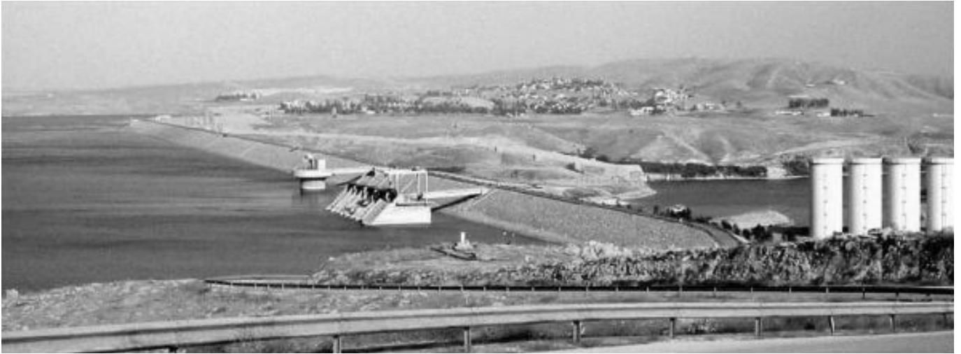
Fig. 2.10 The Mosul dam, 2011, Completed in 1984, the dam suffers from structural problems that caused the U.S. Army Corps of Engineers to once call it 'the most dangerous dam in the world,' an accusation rejected by Iraqi authorities.
