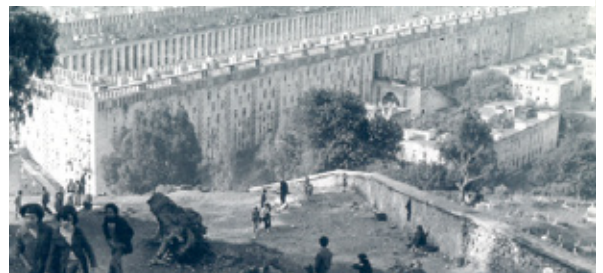
Fig. 4.67 general view of 200 columns
