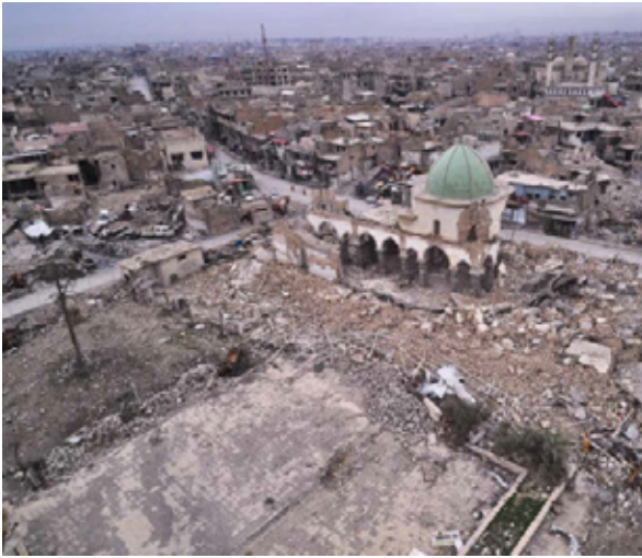
Fig. 1.26 Drone View of Al Nouri Complex after its destruction in 2017.
