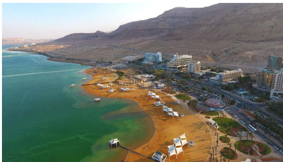
Figure 505. Aerial View of the Dead Sea Promenade. Source: Shlomo Aronson Architects
