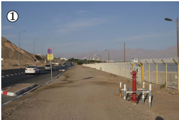
Figure 432. Current situation of the walkway aside the Katza oil, 2024. Source: Author
