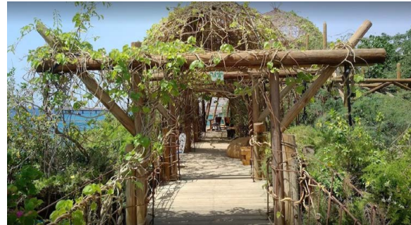
Figure 469. Wooden structure covered with plants
