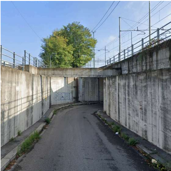
Figure 41. The only entrance to the Via Bonfadini camp via a passageway. Source: street view snapshot (2026).
