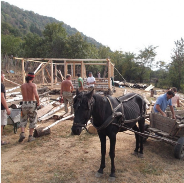
Figure 24. Construction of Odaia (2013) by aaa, as part of the laboratory 'Nomadic School', co-designed and co-built as collective building for eco-tourism, run by a local association to strengthen the local economy and collective governance in the Calinesti area, near the small town of Brezoi in the Romanian Carpathians. Source: Atelier d'Architecture Autogeree (2015).
