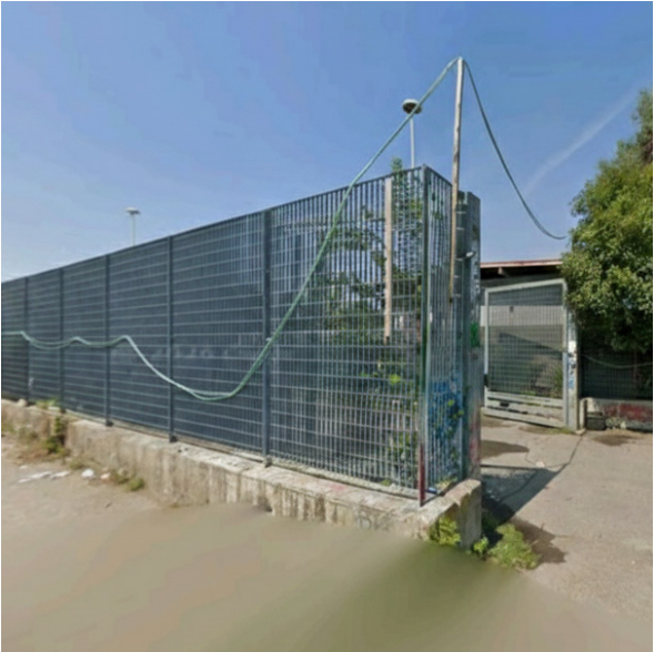
Figure 36. Entrance B and fences of via Chiesa Rossa. Source: street view snapshot (2026).
