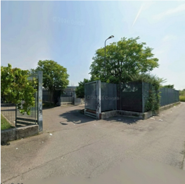
Figure 35. Entrance A and fences of via Chiesa Rossa. Source: street view snapshot (2026).
