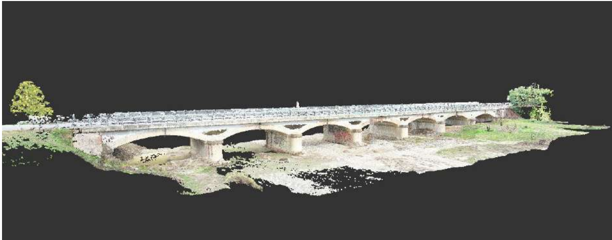
Figure 3.8: Point cloud by Photogrammetry. Font: Autor.
