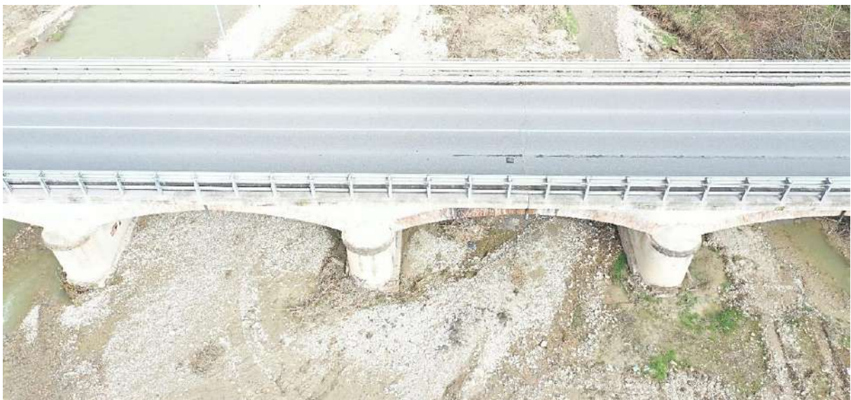
Figure 3.2: Top view of the bridge.
