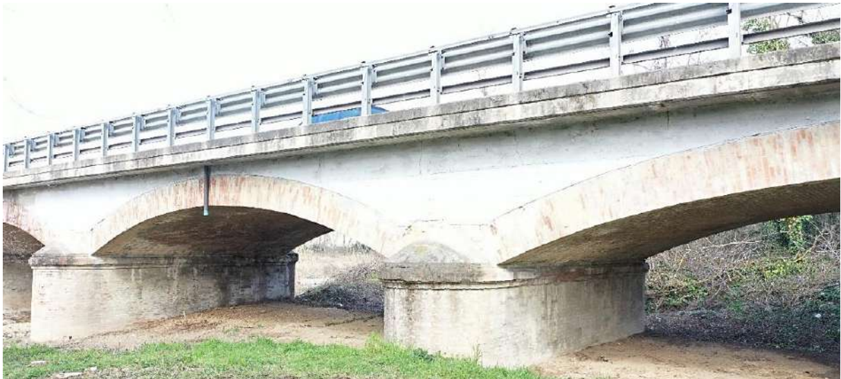
Figure 3.1: Lateral view of the bridge.
