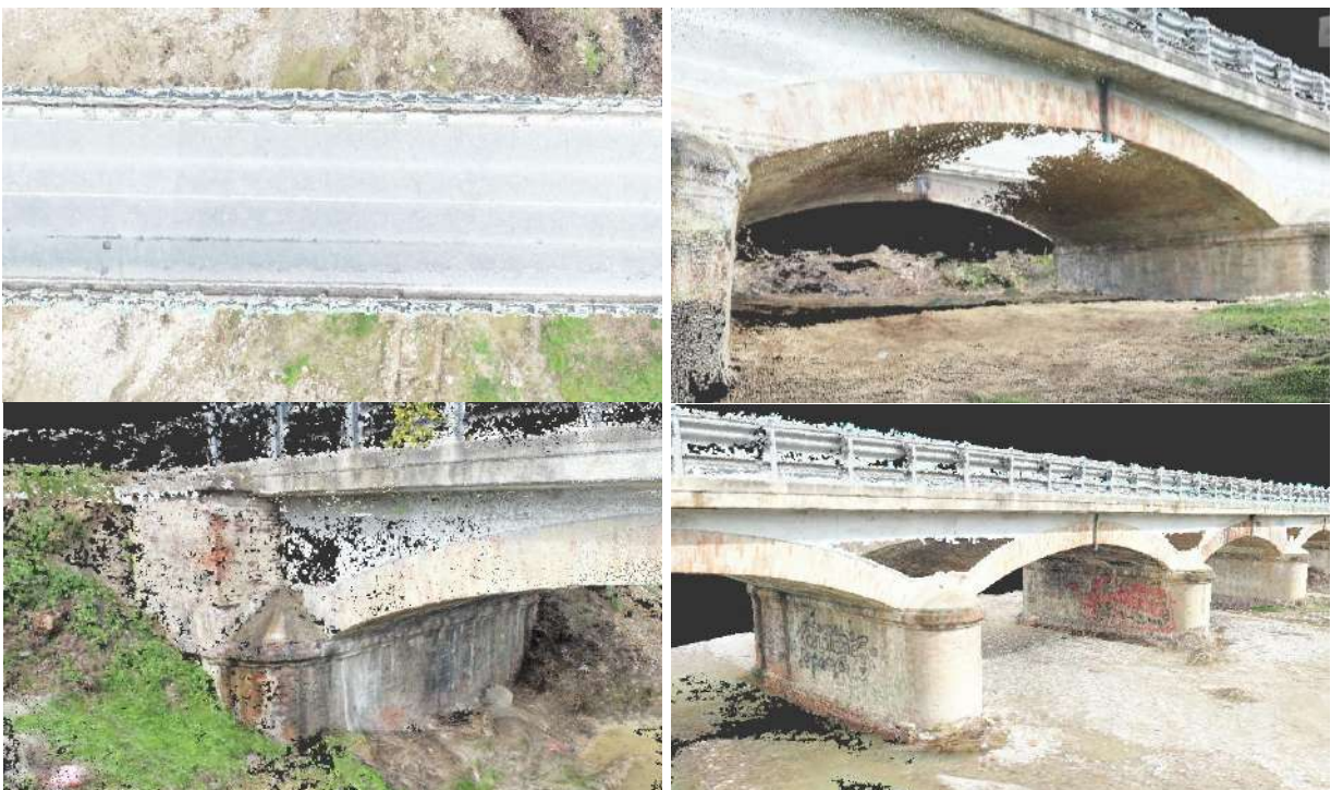
Figure 3.10: Details of the point cloud provided by the drone. Font: Autor.
