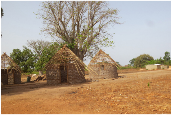
Construction of adobe houses in the Tanaff valley @Balouo Salo
