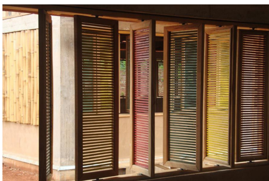
Fig. 8.30 - Colourful bamboo louvres at the Dwabor Kindergarten @ARUP
