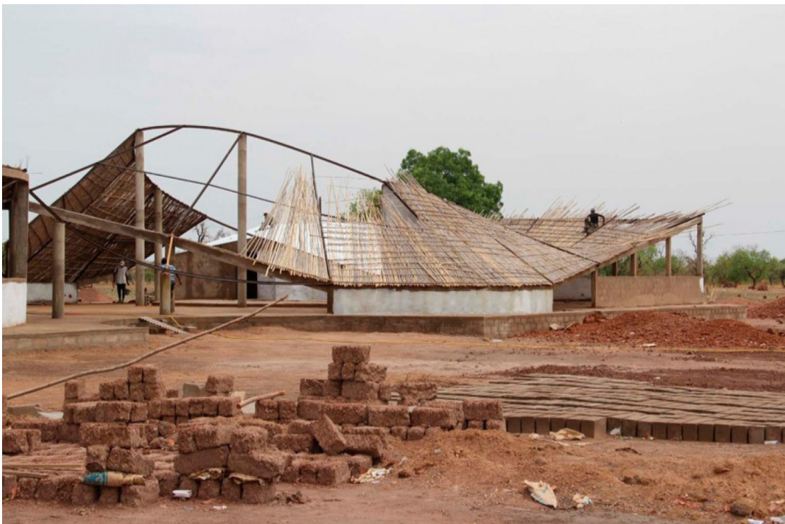
Fig. 5.6 - Fass school under construction @Toshiko Mori Architect
