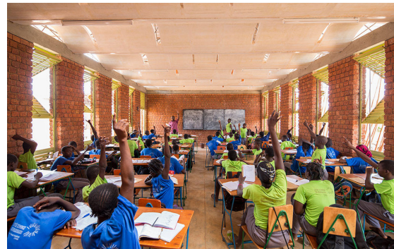
Fig. 1.43 - Classroom with adaptable louvers to provide good lighting @Kere Architecture
