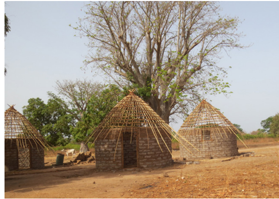
Fig. 2.10 - Construction with adobe bricks and thatch roof @Balouo Salo
