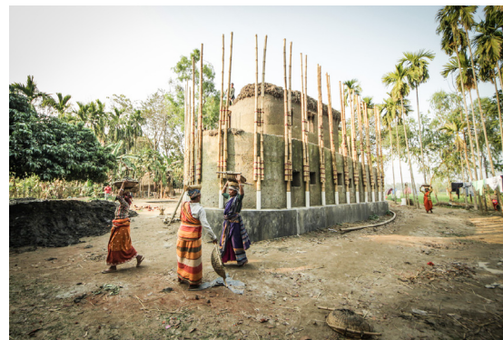
Fig. 5.10 - Construction in progress @S. Mori
