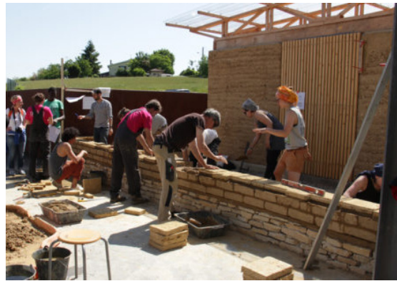
Fig. 3.22 - Community participation on a construction site @AMACO
