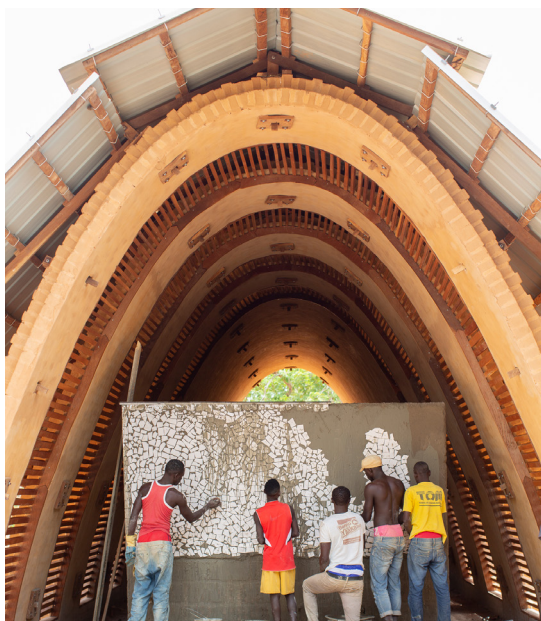
Fig. 5.22 - Construction in progress @J.Valera
