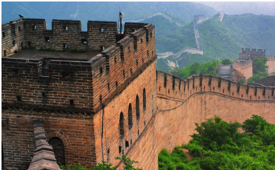
Fig. 3.4 - Portion of The Great wall of China made in clay bricks @ootravels.
