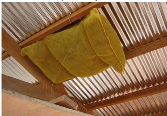
Fig. 5.37 - Coconut husks as isolation @ARUP
