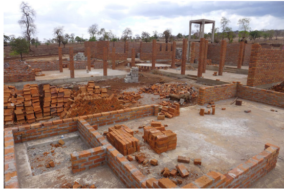
Fig. 5.41 - Construction in progress @Asante
