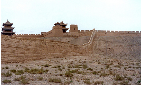
Fig. 3.3 - Portion of The Great wall of China made in rammed earth @Wikipedia
