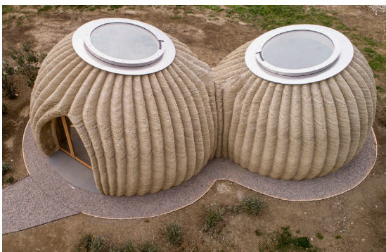
Fig. 3.1 - 3D printing round houses in raw earth in 200 hours @TECLA
