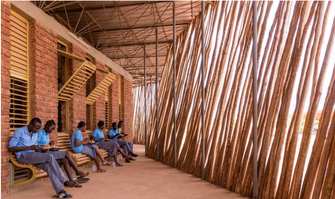
Fig. 5.30 - Porche created by lateral wood lattice @A. Maretto
