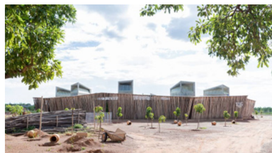
Fig. 8.15 - Solar chimneys on the Lycée Schorge by Kere architecture @I.Baan
