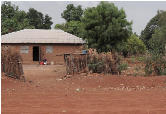
Fig. 2.26 - House made of adobe blocks with a metal roof in Tanaff @Balouo Salo
