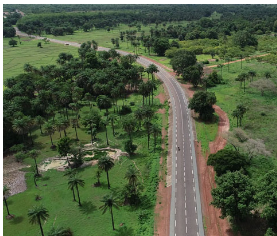
Fig. 1.17 - New regional roads in Sedhiou @Eiffage Senegal
