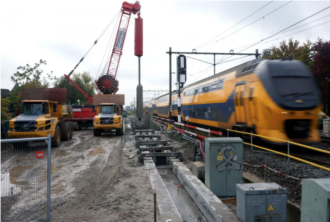
Figure 2.1: Cement Bentonite in-filled trench construction phase [56].
