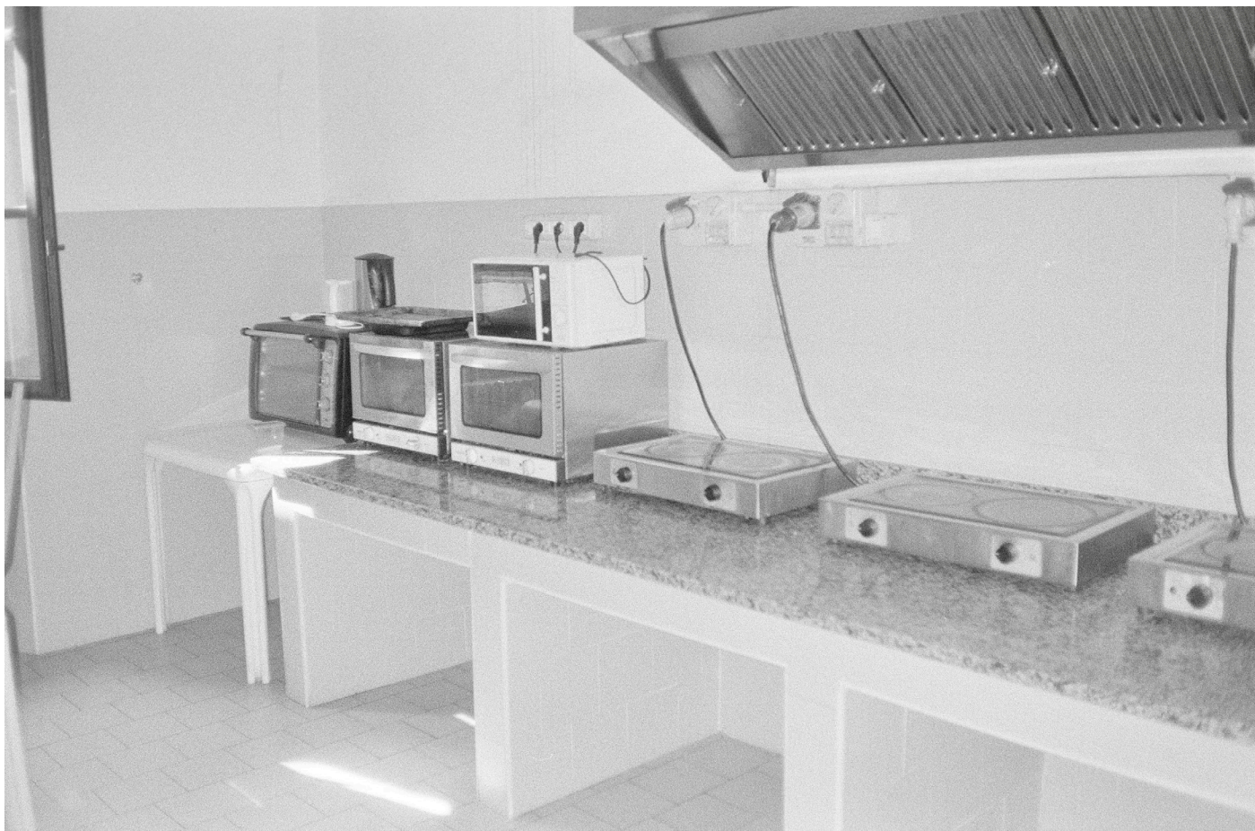
Image 15 & 16. Collegio Cairoli kitchen room. Consisting on a series of electric stoves, the open space allowed students to meet during the pandemic due to the need of cooking outside of rooms. This was the case of many colleges with shared kitchens (author own picture)
