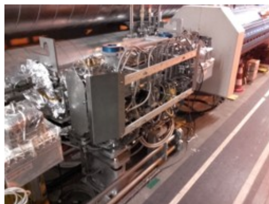
(b) A TCPPM installed in the tunnel
