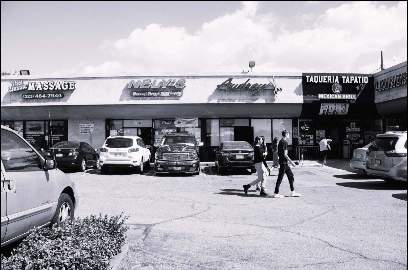
Strip Mall in Los Angeles, USA Figure 13
