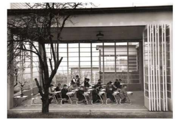
Suresnes Open-Air School Marcel Lods, Eugène Beaudouin, 1935
