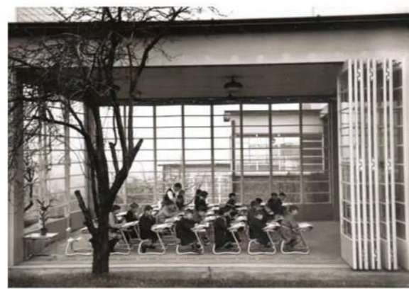
Suresnes Open-Air School Marcel Lods, Eugène Beaudouin, 1935
