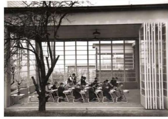
Suresnes Open-Air School Marcel Lods, Eugène Beaudouin, 1935
