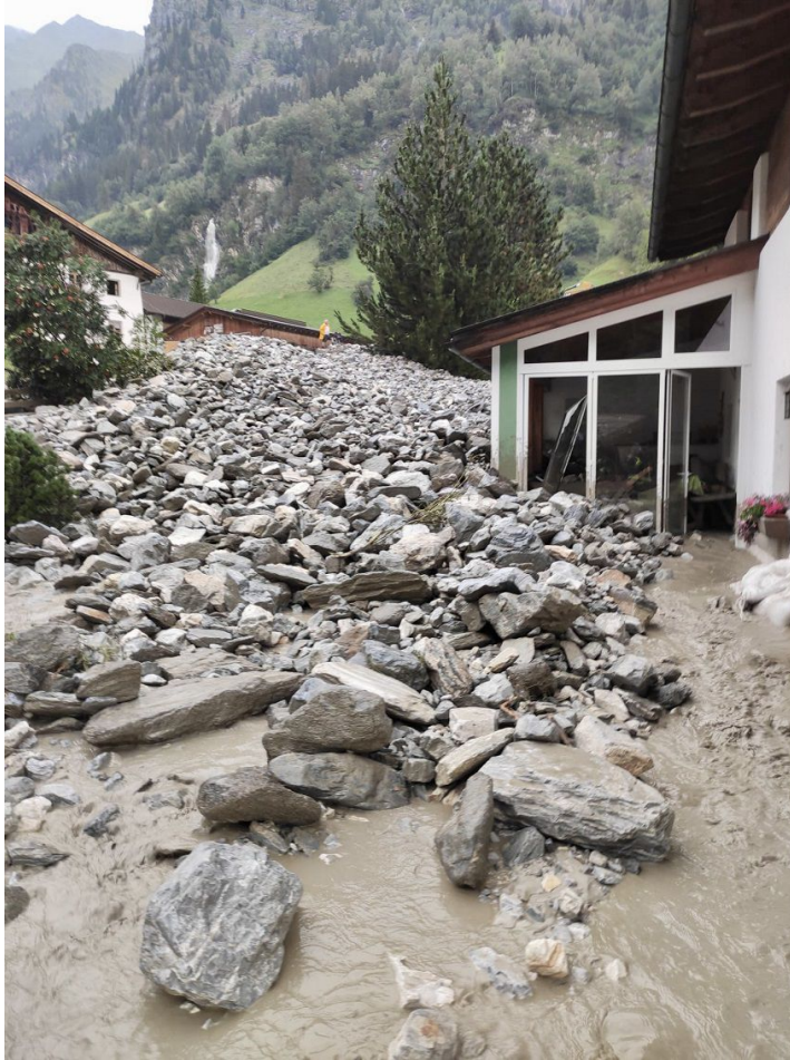
Figure 1.7: Debris flow damage in South Tyrol region [10]
