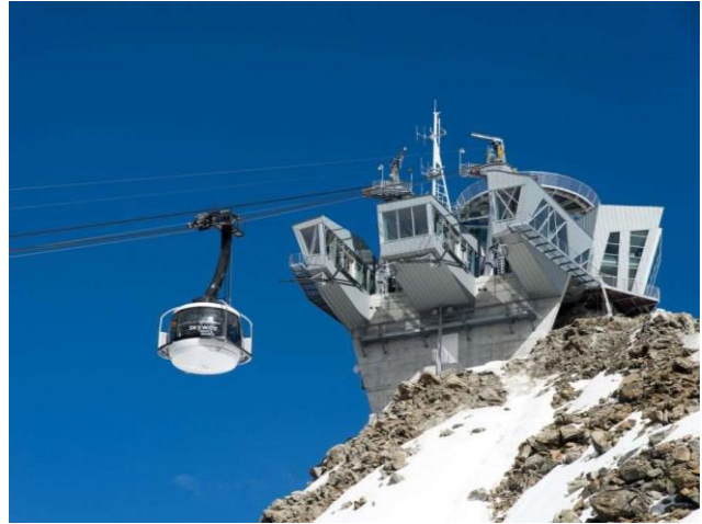
Figure 4.2 Upstream station of Punta Helbronner. Source: https://sertec-engineering.com/blog/skyway-monte-bianco/
