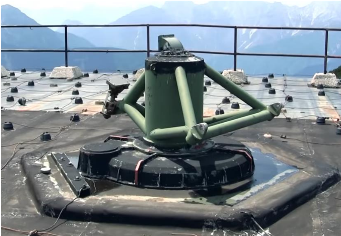
Figure 2.15 The remaining rotating support with the waveguide.
