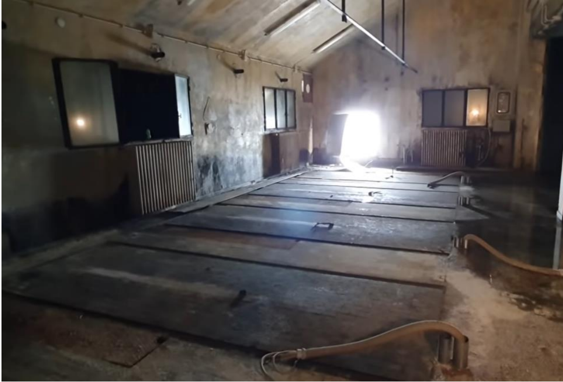
Figure 2.6 The power station of the military site in the upstream station.
