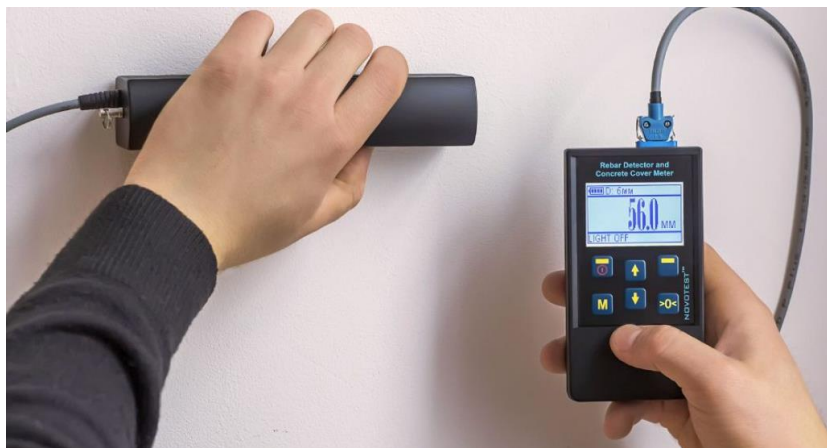
Figure 4.9 Pacometer test. Source: https://www.structuralsurveys.it/indagini-su-strutture-in-calcestruzzo-prove-pacometriche/
