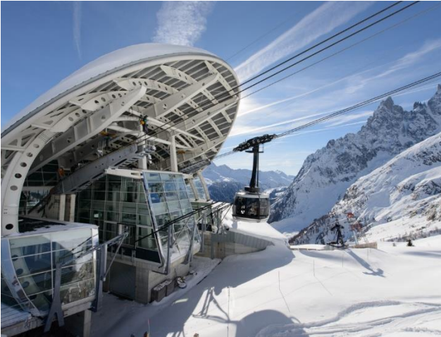
Figure 4.1 Intermediate station of Pavillon du Mont Frèty. Source: https://www.h-b.it/it/portfolio-view/mont-blanc-pavillon-du-mont-frety-funivia-courmayeur-ao/
