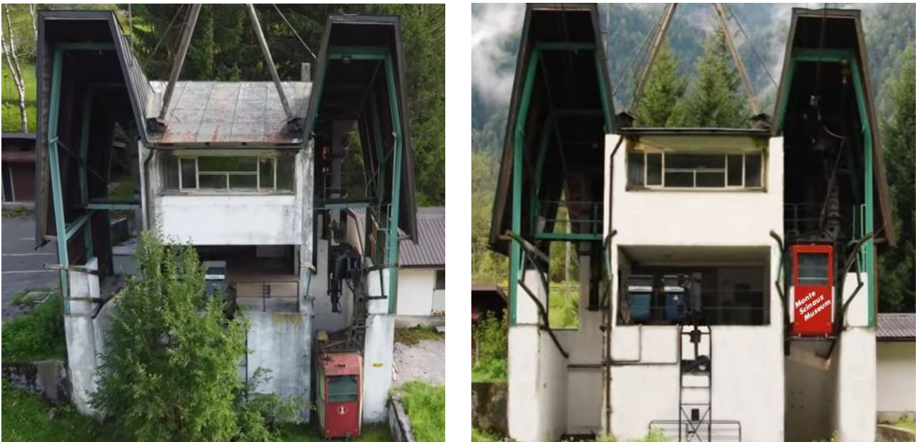
Figure 4.12 Downstream station before and after refurbishment interventions.
