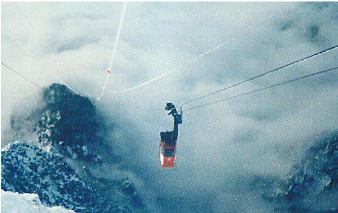
Figure 2.2 Photograph of Monte Scinauz Cableway in operation during winter months.
