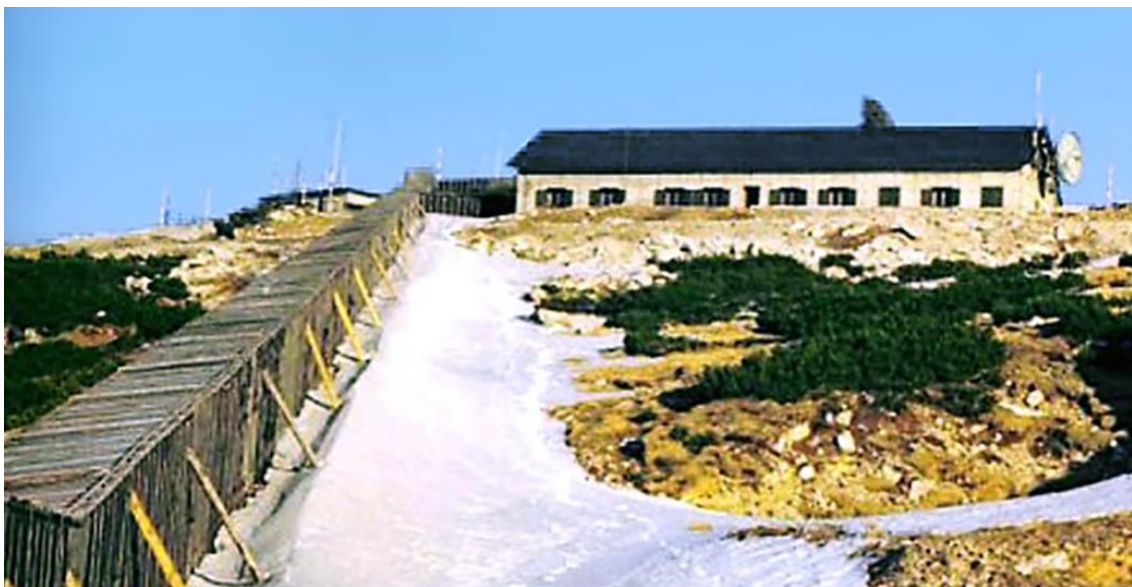
Figure 2.10 The old tunnel in wooden structure.
