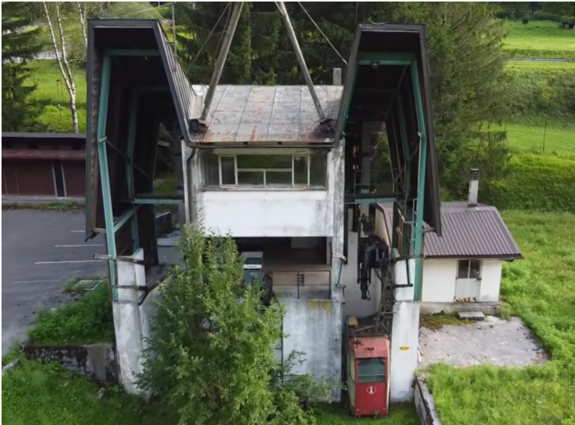
Figure 2.4 Downstream station of Monte Scinauz Cableway.
