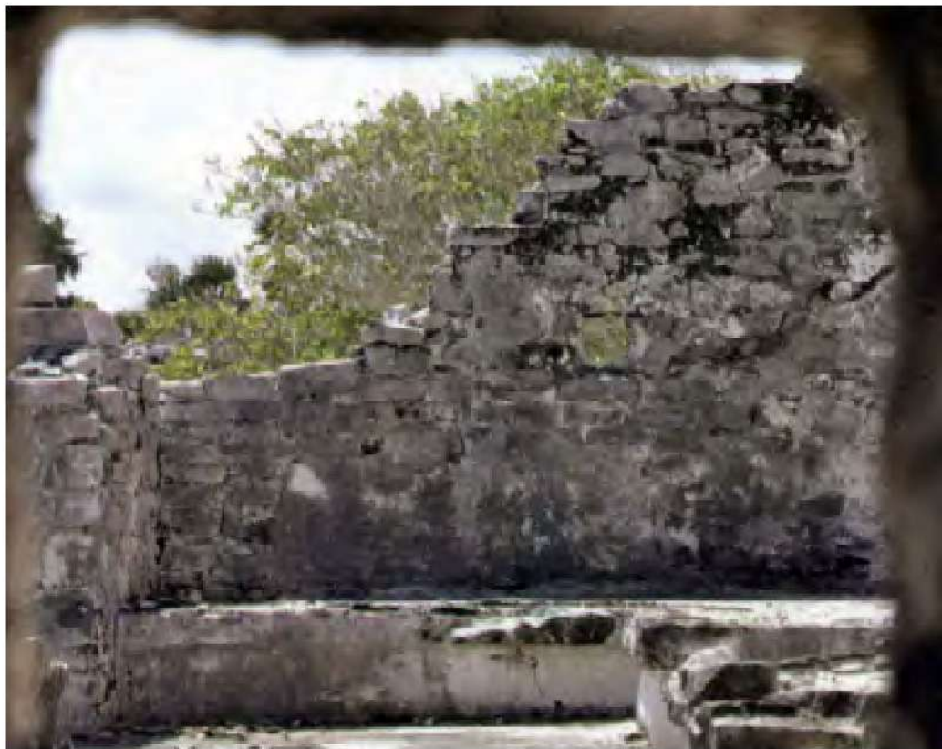
30. Structure 25 seen to the west through the holes in the east and west walls of the south anteroom: note the height of the western hole with respect to the segment of the wall visible in the background on the left. Photo by: Ivan Sprajc
