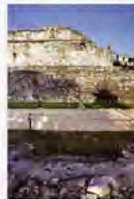
West façade of structure 25, looking from the stairway of structure 29 to the east
