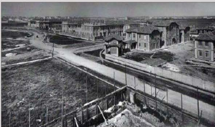
ARIEL VIEW OF POLIMI AND UNIMI AGRARIA BLOCK CONSTRUCTION PHASE
