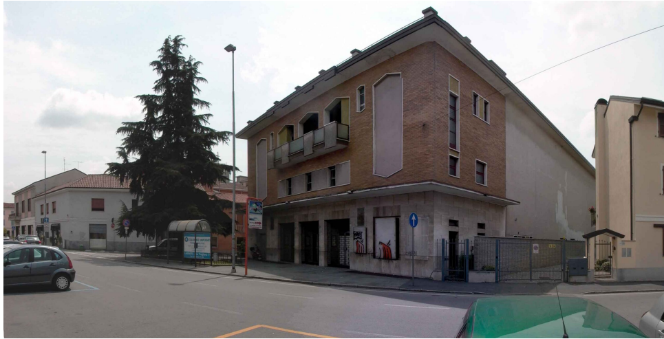
Figure 1: State of fact of the old cinema located in Lainate to be requalified.
