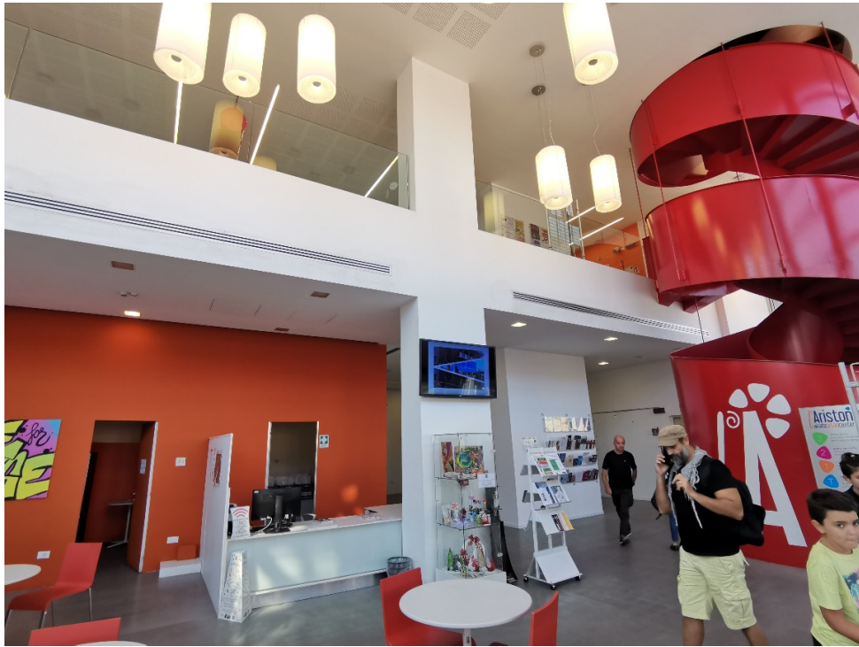
Figure 4.9: Linear diffuser in the atrium.
